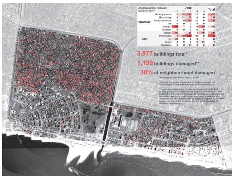
Source : UNITAR-UNOSAT (2019), Mozambique Chipangara Neighbourhood / Cidade da Beira Distrito / Sofala Province Imagery analysis: March 26 2019 | Published March 28 2019 | Version 1.0 Figure 5-9 Damaged facilities in the event of Cyclone Idai (Chipangara Bairro)
