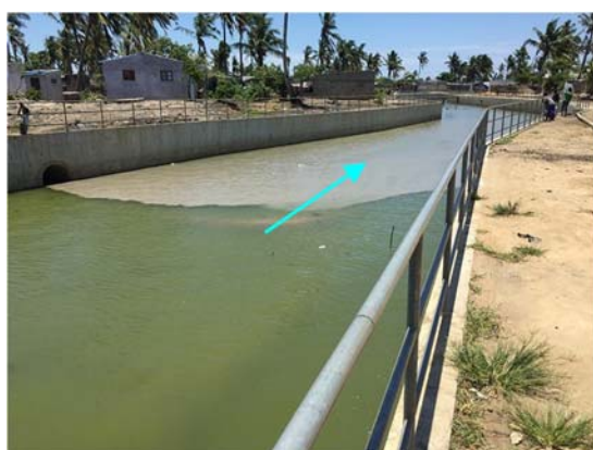
(1) No damage to the channel
