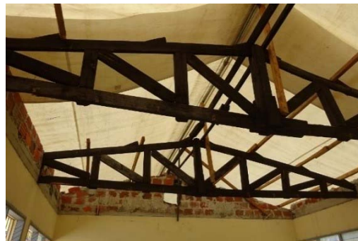
Internal Appearance of Temporary Roof
