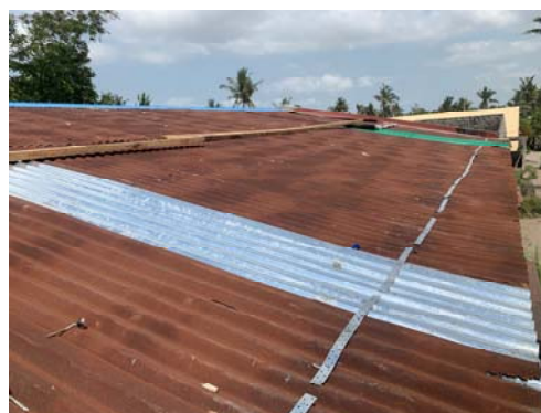
(b) Rehabilitated Roof
