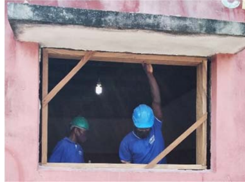
(b) Installation of Window Frames
