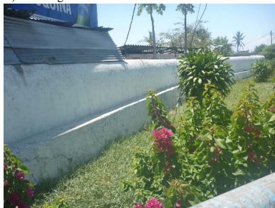
D) No damage to the old seawalls
