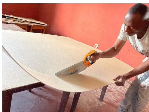
(c) Cutting out the new ceiling sheets
