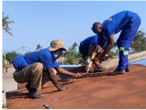
(b) Rehabilitation on the Roof
