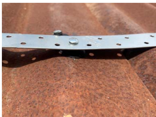
(a) Reinforcement by Metal Band
