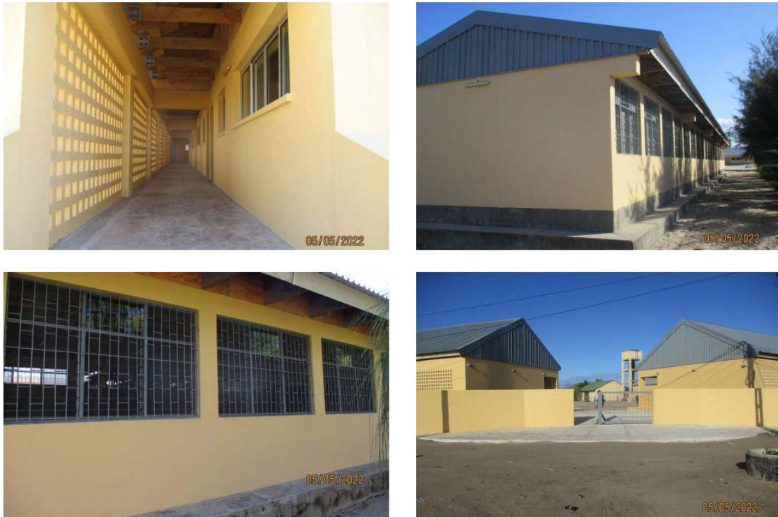
Figure 9-14 EPC Macurungo / Site photo (after rehabilitation)
