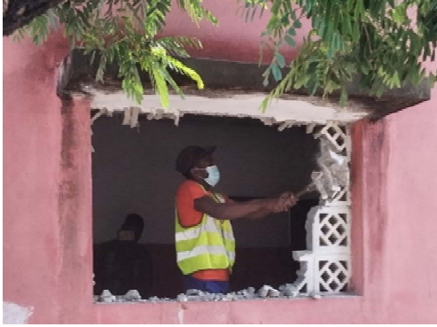
(a) Removal of Bricks
