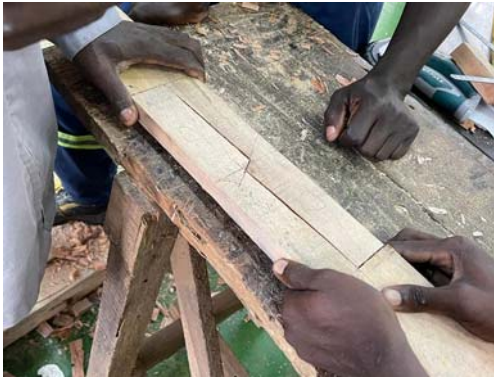
(h) Processing the Joints (Day 3-4)
