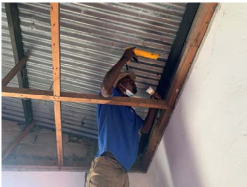
(c) Rehabilitation from inside
