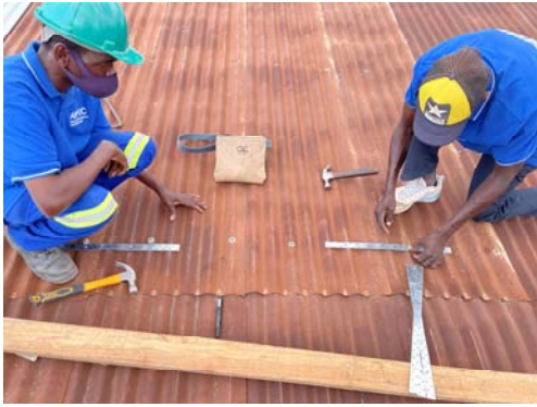
(a) Rehabilitation on the Roof
