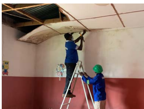
(a) Removal of Existing Nails and Ceiling Sheets
