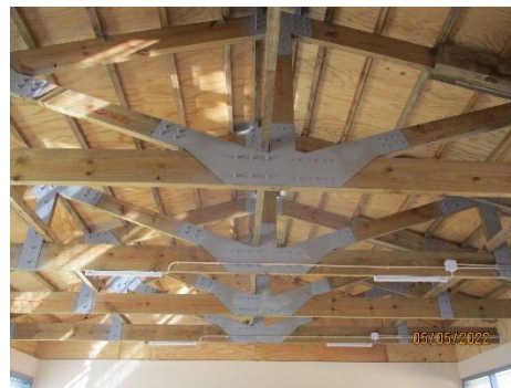
The Roof was Rehabilitated in a Resilient Way
