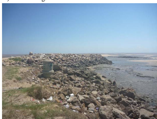
F) No damage to the jetty at the estuary
