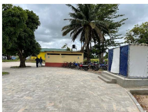
Paved Plaza Constructed
