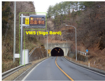
VMS (Sign Board)
