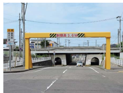
Figure 8.2.15 Height Restriction Barrier
