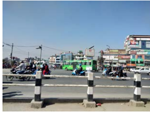
Source; JICA Survey Team Figure 8.2.17 Existing Railings
