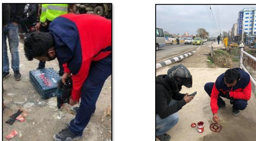
Figure 3.1.2 Benchmark Installation
