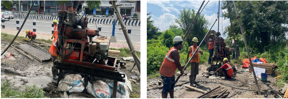
Photo 3.3-1 Core Drilling
