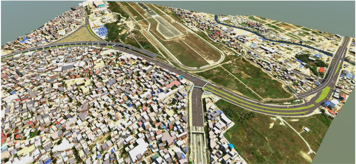
View-01 Overview of the Project
