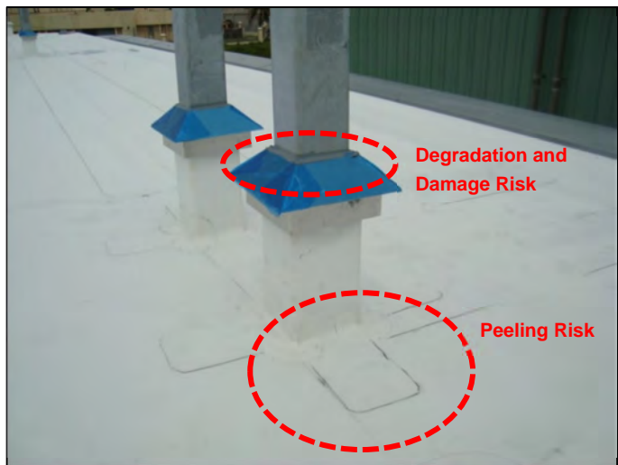
Figure 1-4: Photo of Pillar Construction
