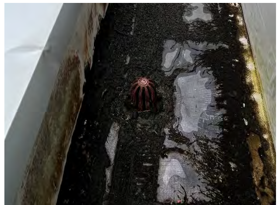
Condition of Existing Roof Drain
