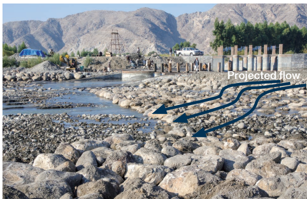
Photo 7.8 Ingenuity to Reduce the Water Force from the Top of the Weir 1)
