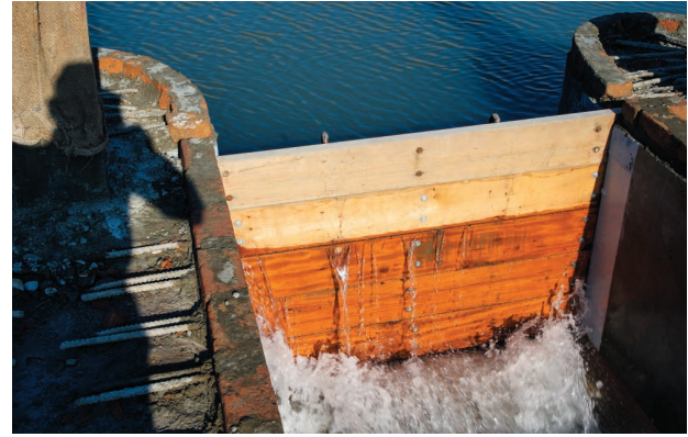
Sand Flushing Ditch
