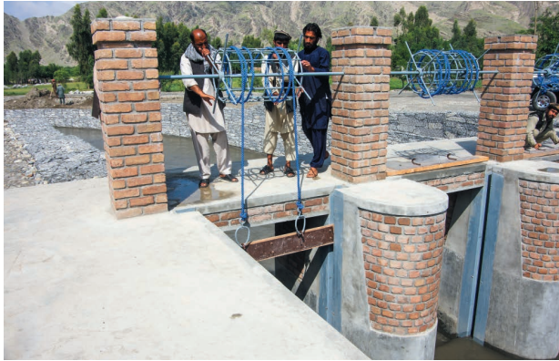
Inspection of Intake Gate
