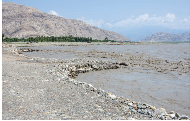
Photo 7.11 Reinforcement of Riverbanks and Correction of Streamway by Installing Spur Dikes 1)
