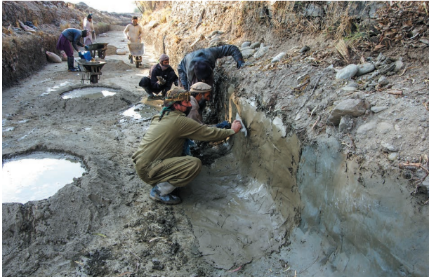
Lining Situation in an Irrigation Canal
