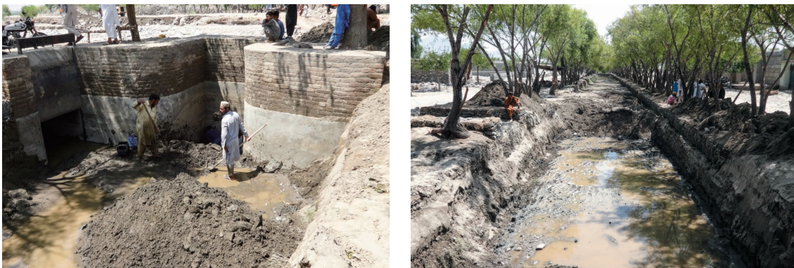
Photo Extended Flood Crossing Bridge 1)
