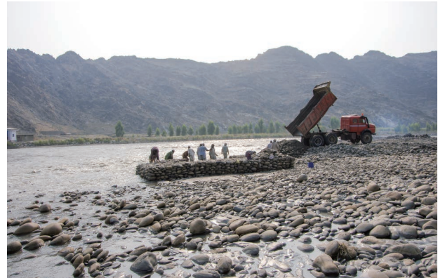
Photo 7.7 Restoration of Sandbar by Gabion Works 1)
