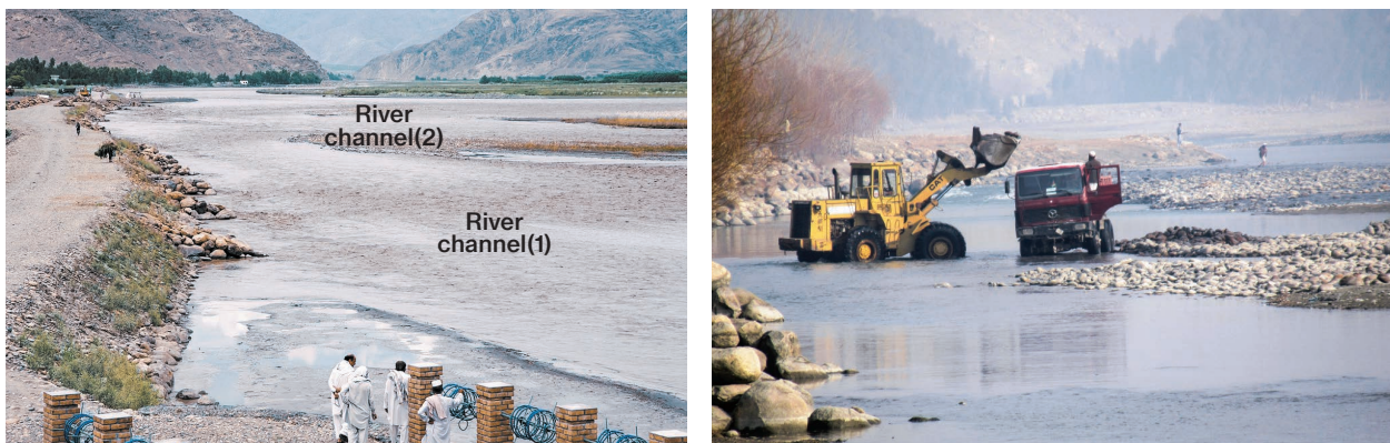
Photo 7.12 River Channel Excavation and Sediment Dredging at Miran Weir 1)
