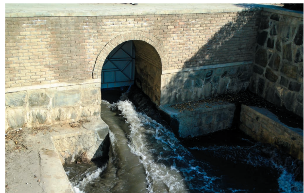
Drainage Gate (outflow)
