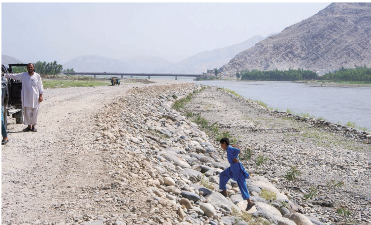
Photo 6.53 Riprap Works on the Riverside Dike Slope (Behsud Bank Protection) 1) : June 18, 2011
