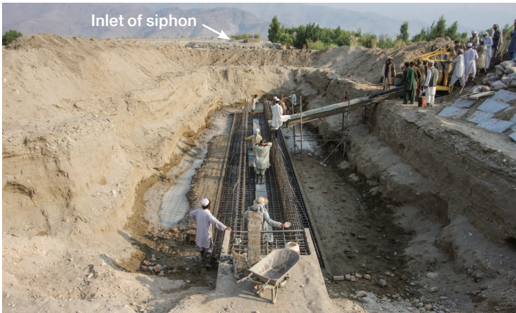
Photo 6.43 Construction of a Siphon (Marwarid Canal, Gamberi Floodway) 1) : October 24, 2012
