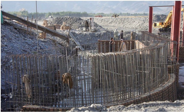
Photo 6.18 Reinforcement of Concrete Revetment (Kashkot Intake Gate) 1) : November 7, 2012
