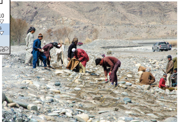
Figure 5.10 Strengthening Dikes by Planting Trees 1)
