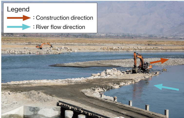
Photo 6.5 Locating the Oblique Weir with Boulders (Marwarid Weir II) 1) : October 16, 2018
