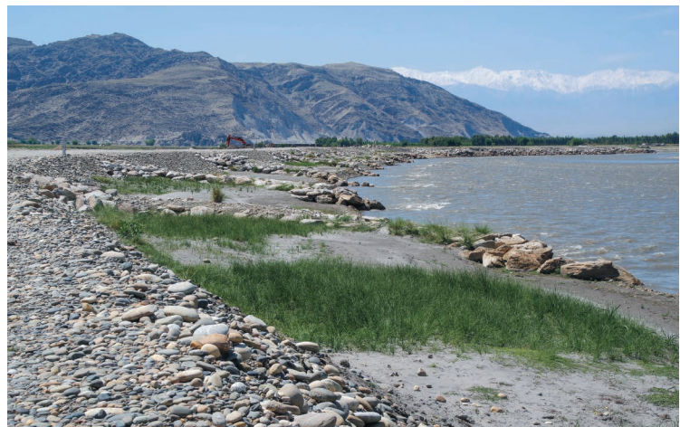
Figure 5.15 L-Shaped Spur Dikes 1)
