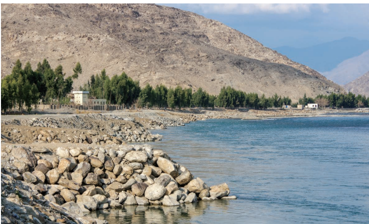
Photo 6.57 Construction of a Group of the Stone Spur Dikes (Miran) 1) : January 24, 2015
