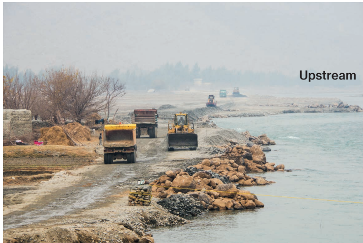
Photo 5.3 Dike Crown utilized as Access Road 1)
