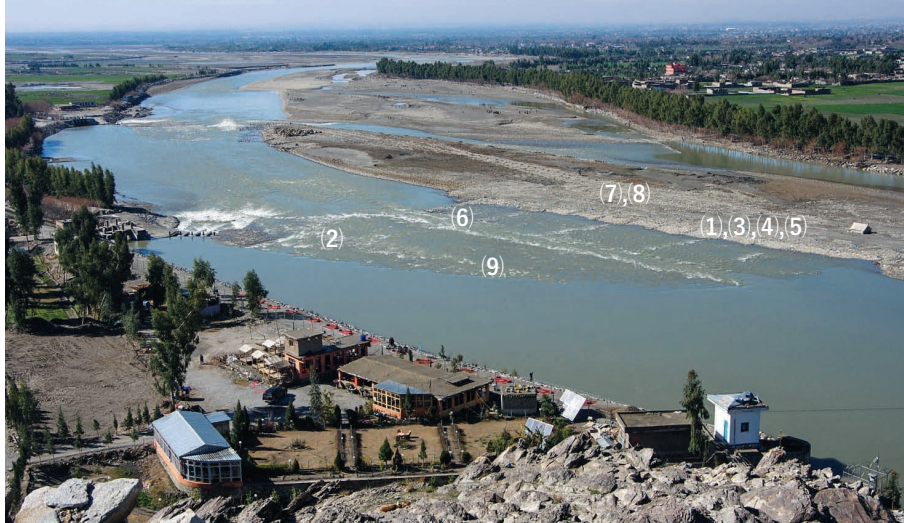
Note: Numbers in parentheses correspond to those of each construction process below.
