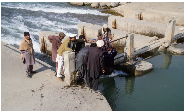
Photo 6.23 Flush Board Removing Test (Marwarid Weir II Sand Flushing Ditch) 1) : January 22, 2019
