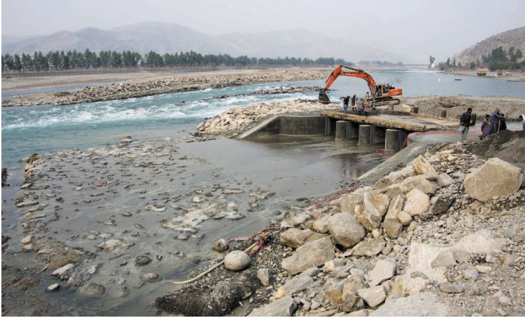
Photo 6.24 Apron and Downstream Bed Protection of the Sand Flushing Ditch (Kama Weir II Sand Flushing Ditch) 1) : January 17, 2018
