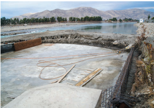
Photo 6.3 Cofferdike(Cutoff Wall, Kama I) 1)
