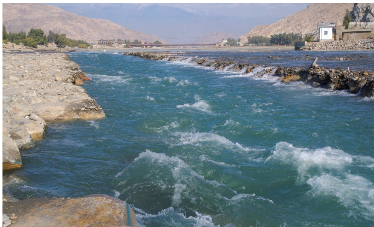
Photo 6.10 The State of Water Flow in Spillway (Kama Weir I) 1) : December 24, 2018
