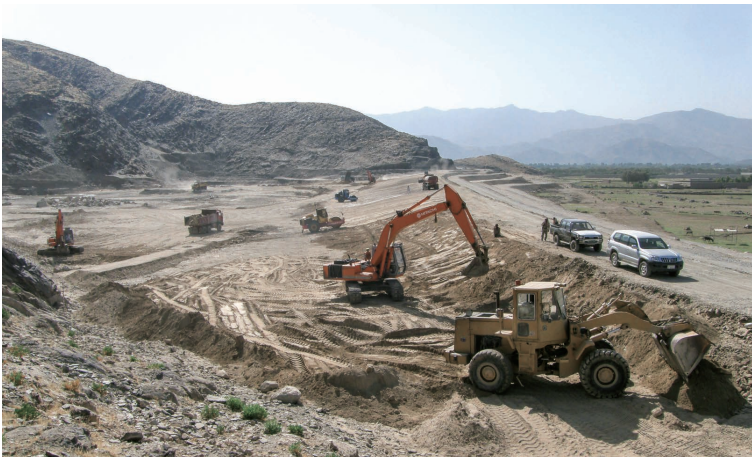
Photo 6.28 Blanket Works (Marwarid Main Irrigation Canal Q2 Reservoir) 1) : July 15, 2009
