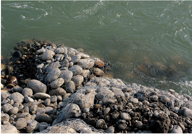
Photo 5.2 Foot Protection Works applying Combined Gabions 3)
