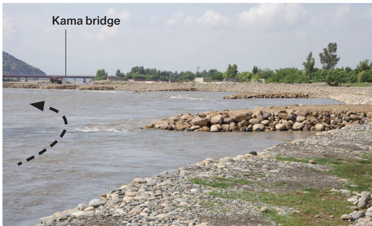
Photo 6.58 River Flow at Installation Section of Stone Spur Dikes at the Curved Part Where Erosion is Most Intense (Miran) 1) : April 20, 2015
