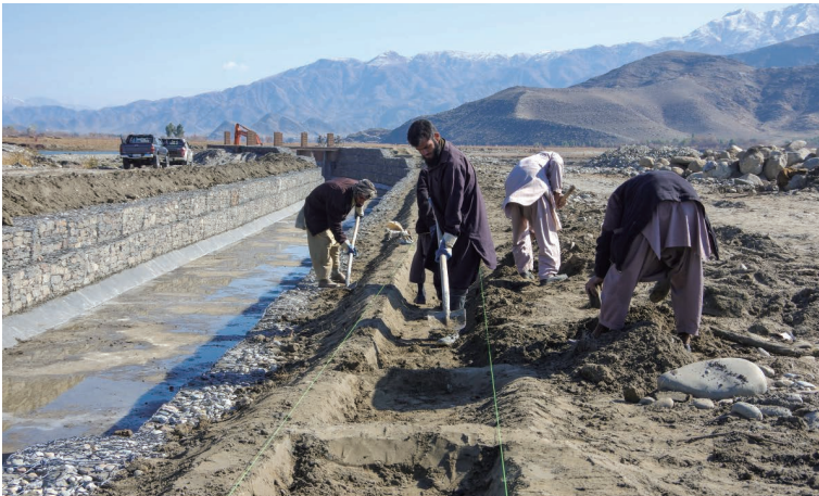
Photo 6.37 Making Ridges prior to Wicker Works (Shigi Main Irrigation Canal) 1) : January 29, 2015
