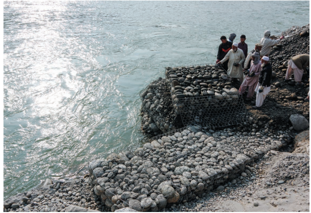
Photo 5.2 Foot Protection Works applying Combined Gabions 3)
