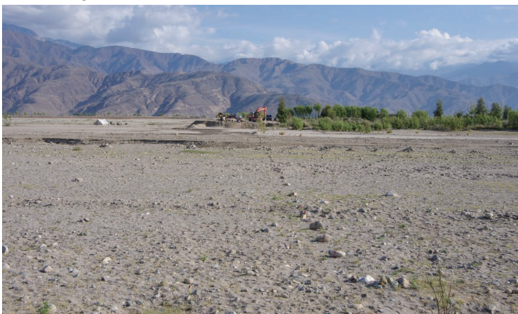
Photo 6.42 The Status before Constructing the Siphon (Marwarid Main irrigation Canal, Gamberi Floodway) 1) : April 10, 2012
