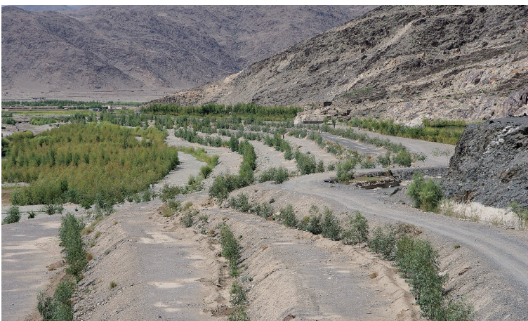
Photo 6.29 Strengthening back slope of the Reservoir Embankment by Eucalyptus (Marwarid Main Irrigation Canal Q2 Reservoir) 1) : September 19, 2011
