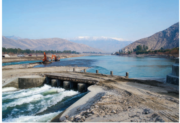
Photo 6.2 Example of a temporary bridge (Kama weir II) 1)
