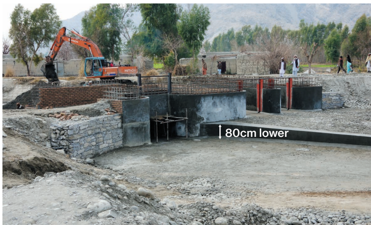
Photo 6.46 Height Difference at the Drain Gate (Miran) 1)
