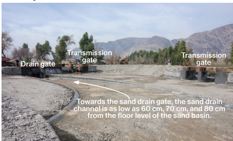
Photo 6.49 The Sand Basin Configuration (Miran) 1)
