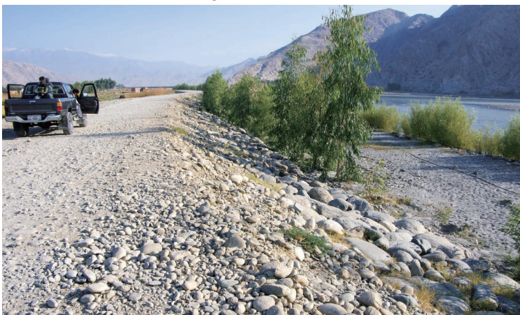
Photo 6.54 Dike Protection by Vegetation Works (Behsud Bank Protection) 1) : October 24, 2012
