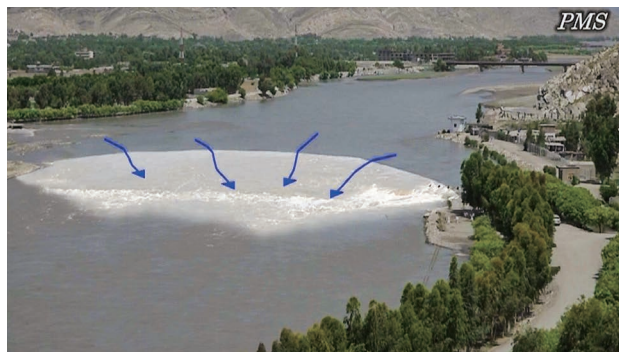
(10) Completion of boulder oblique weir: water can be stably drawn by increasing the water level at the intake weir. (Kama Weir I)
