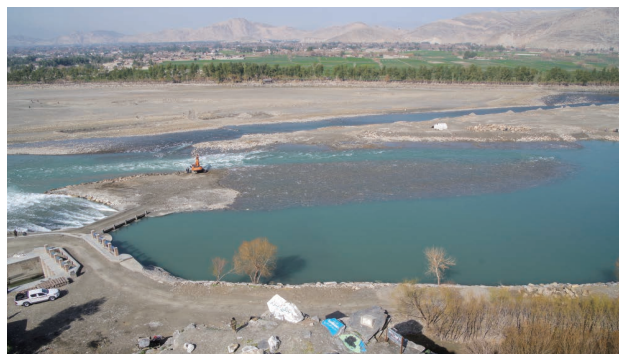
(12) Construction is completed. (Kama Weir II)
