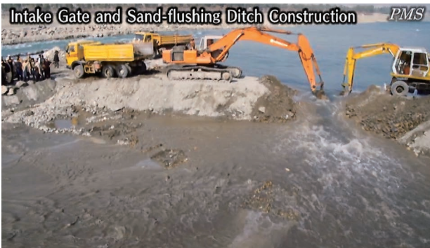
(7) Removing temporary works: after constructing intake gate and sand flushing ditch, remove temporary coffer dike and conduct water into the coffered area. (Kama Weir I)
