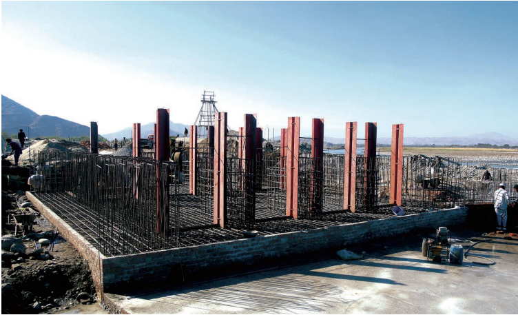
Photo 6.15 Form Works by Bricks (Marwarid II Intake Gate) 1) :November 8, 2016
