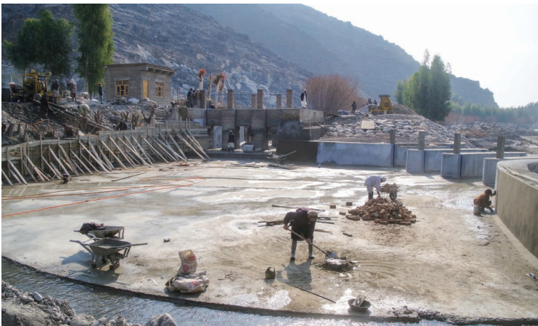
Photo 6.19 Construction of Intake Gate, Sand Flushing Ditch and Sedimentation Pool (Kama Weir I Intake Gate) 1) : January 22, 2019
