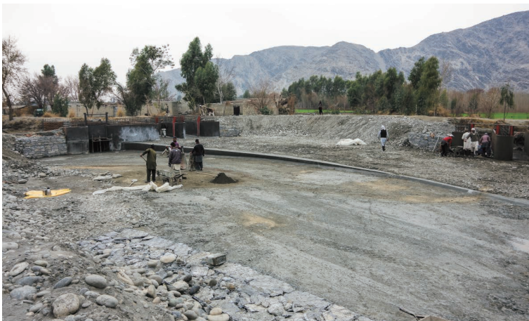
Photo 6.48 Concrete Lining Works in the Sand Drain Channel (Miran) 1) : February 7, 2015
