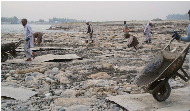
Photo 6.7 Laying out Filling Stones (Kama Weir I) 1) : October 31, 2018
