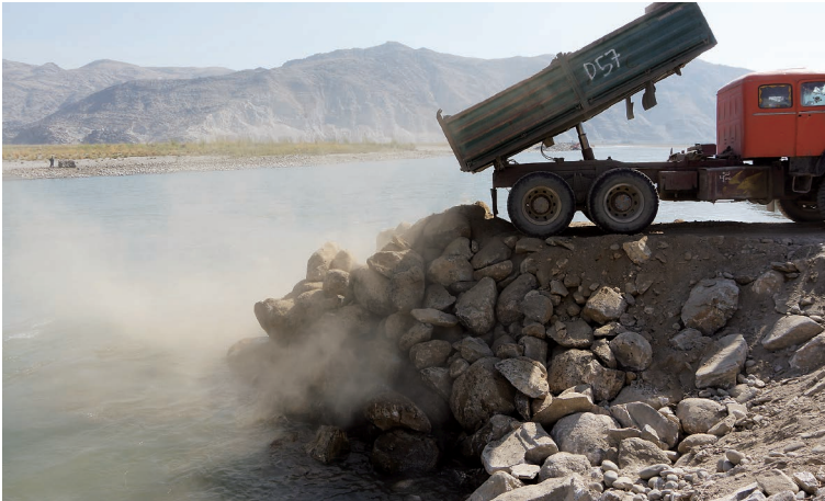
Photo 6.55 Construction of the Stone Spur Dike Foundation (Miran) 1) : October 22, 2014
