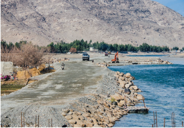
Photo 6.1 Example of a dike using as temporary road (Miran project) 1)
