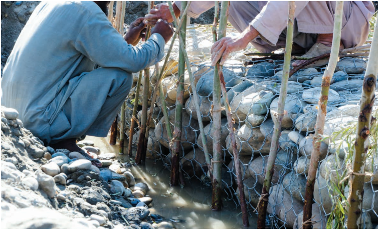
Photo 6.12 Fixing of Wickers (Miran) 1) :October 22, 2015
