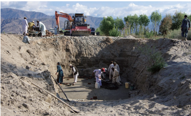
Photo 6.44 Construction of the Siphon Shaft Foundation (Marwarid Canal, Gamberi Floodway) 1) : April 10, 2012
