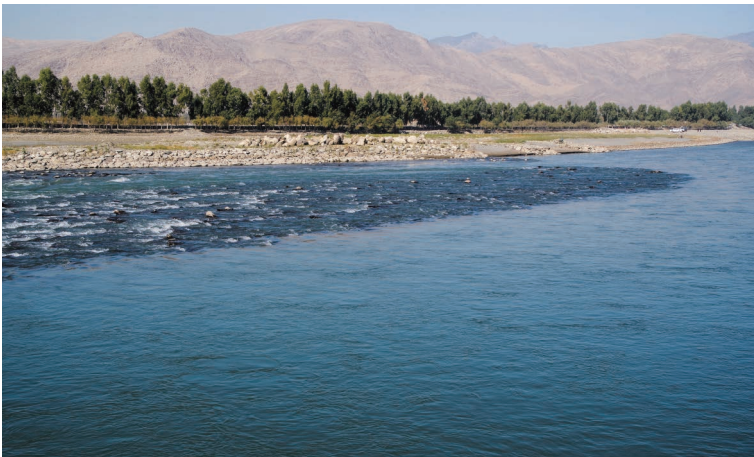
Photo 6.13 Completed Intake Weir (Kama Weir I) 1) :December 1, 2018
