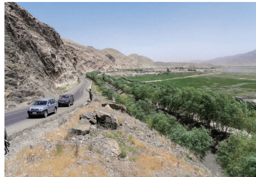
The same location four years after construction. As of May 10, 2009.
