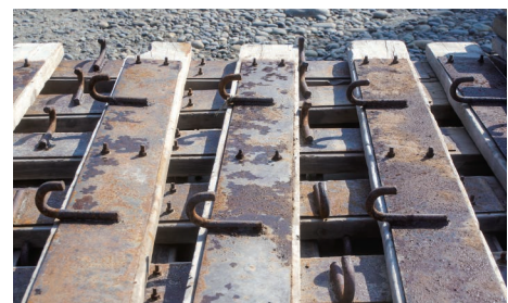
Flush board reinforced by steel plate March 9, 2017
