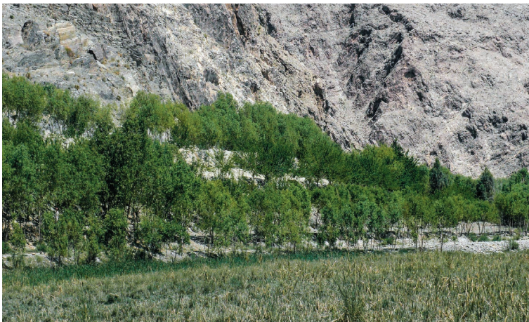
Photo 6.40 Planting on the Back Slope of Canal Embankment (Marwarid Main Irrigation Canal, FG Section) 1) : March 28, 2010
