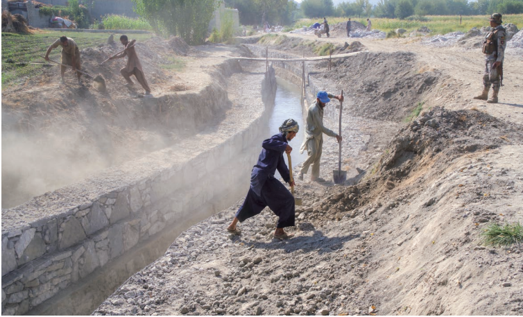
Photo 6.51 Earth Retaining on the Upper Part of the Main Drainage Canal (Gamberi Main Drainage Canal) 1) : September 28, 2017
