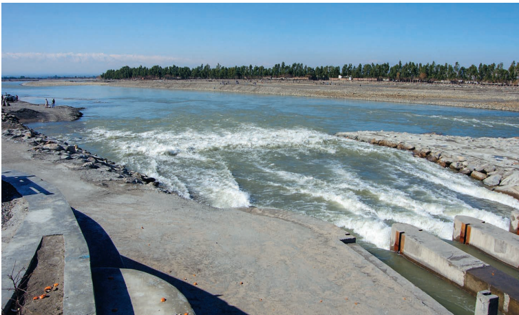
Photo 6.25 Formulation of Apron and Downstream Bed Protection of the Sand Flushing Ditch (Kama Weir II Sand Flushing Ditch) 1)
