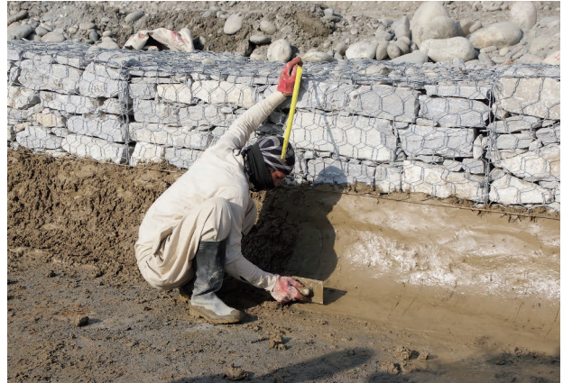
Photo 4.14 Canal Corner Filled by Soil Cement 3)
