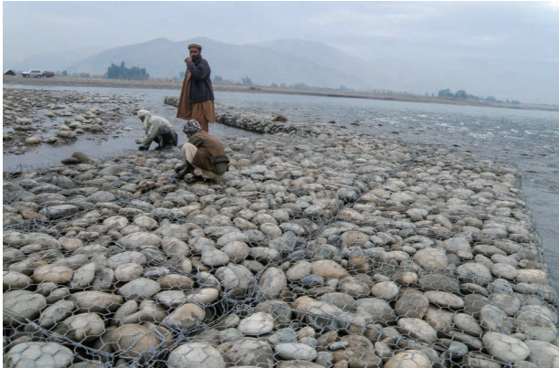
Photo 4.4 Foot Protection Works in the Sand Bar (Kama Weir I) 1)
