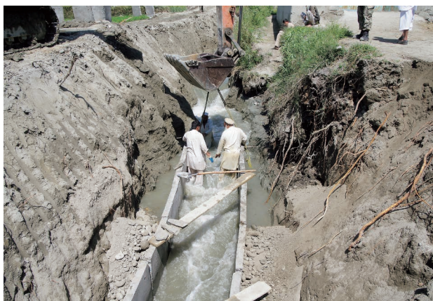
Photo 4.21 Laying the Precast Concrete U-shaped canal 1)
