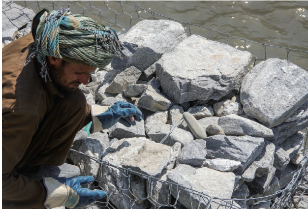
Figure 4.36 How to Fill Stone Materials in Gabion Works 3)
