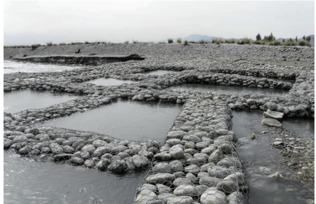
Photo 4.5 Gabion Grid Connection in the Foot Protection Works (Kama Weir II) 1)
