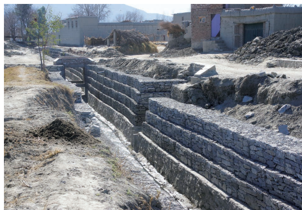
Photo 4.22 Upper Earth Retaining Wall of the Main Drainage Canal 1)
