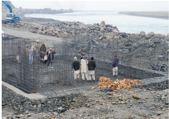
Photo 4.6 Intake Gate under the Construction: constructing a reinforced concrete foundation 1)
