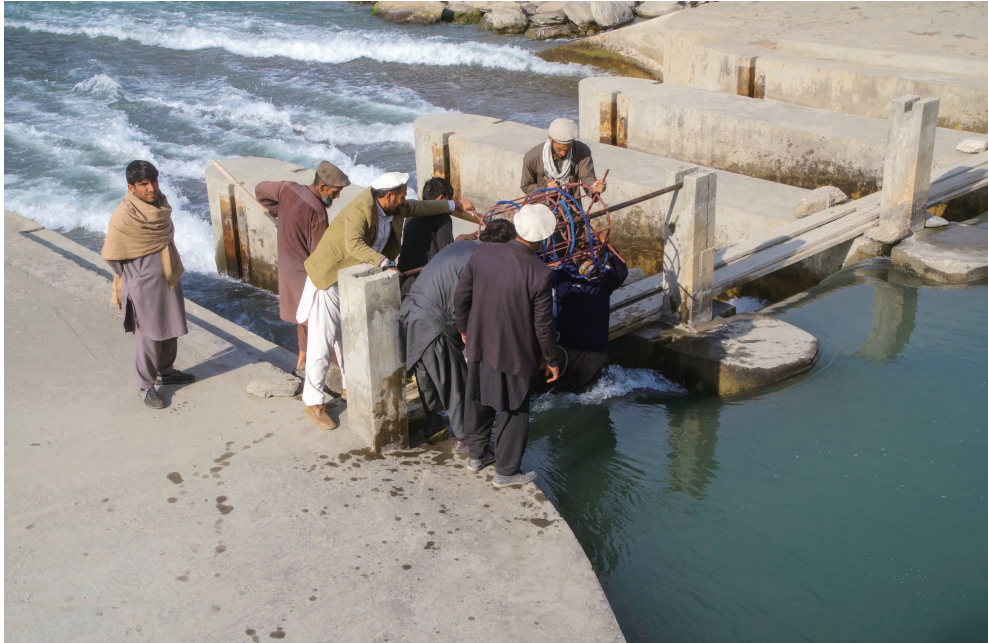
Photo 4.7 Sand Flushing leveraging the Double Flush Boards 1)
