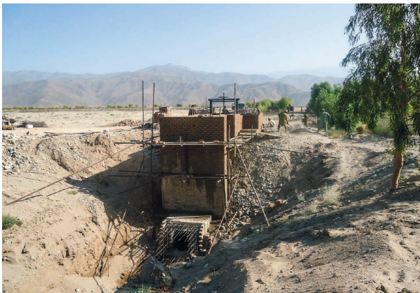
Photo 4.19 The Siphon (under construction) and Flood Crossing Bridge Crossing the Flood Area 1)
