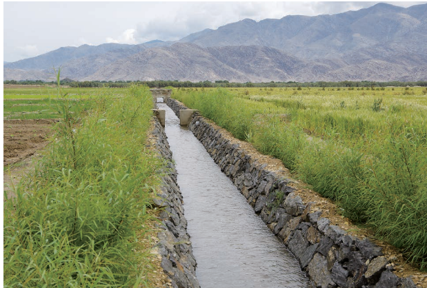
Photo 4.23 Example Stone Masonry for a Small Canal Wall 3)
