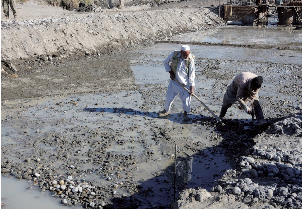
Photo 4.13 Finishing Work by Soil Cement Lining 3)
