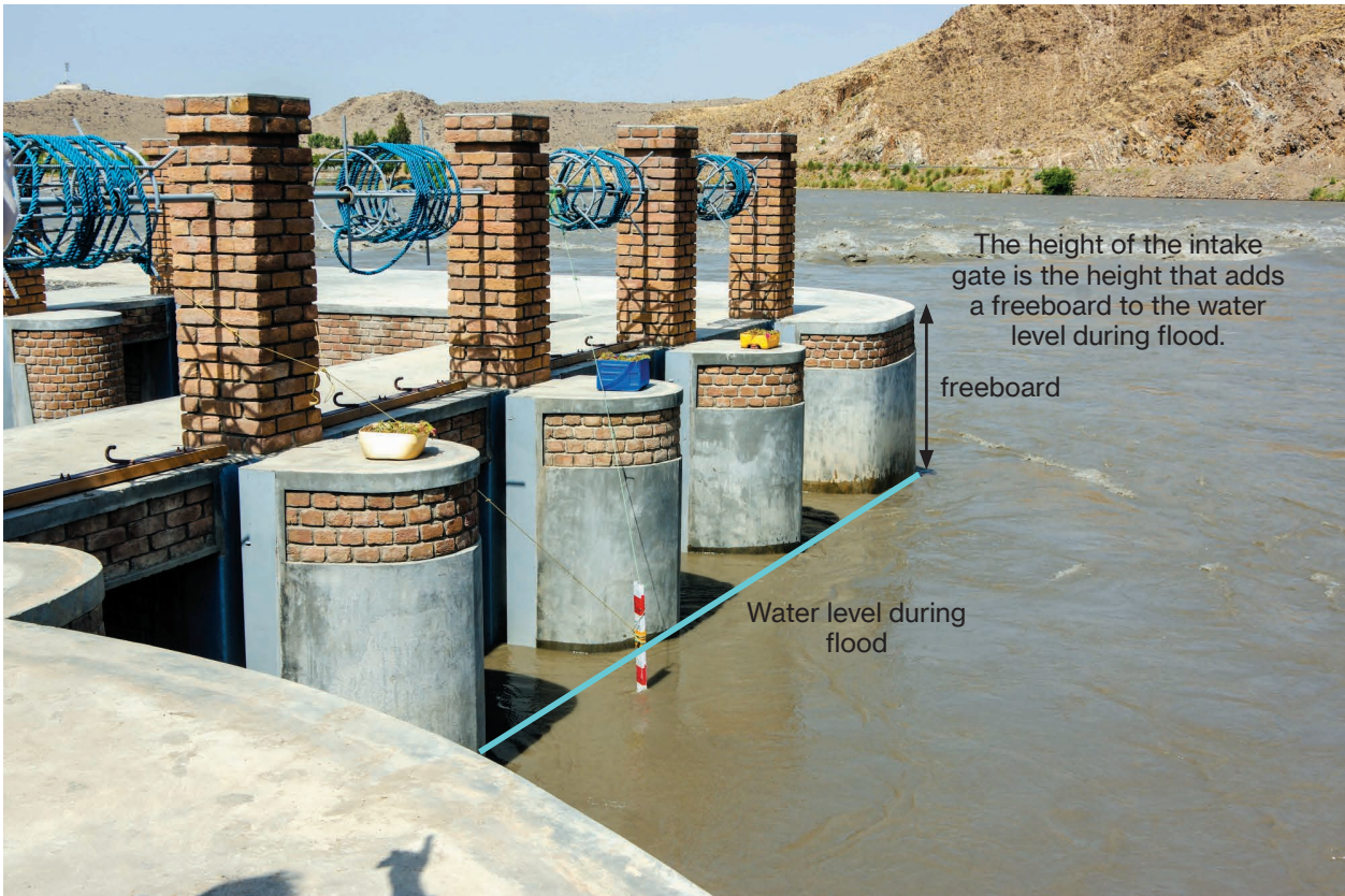
Photo 3.6 Relationship between Water Level During Floods and Height of Top of Intake Gate 1)
