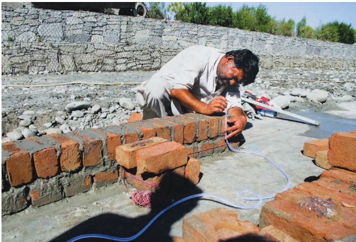
Figure 3.11 Examples of Measuring Distance, Depth and leveling by Simple Surveying
