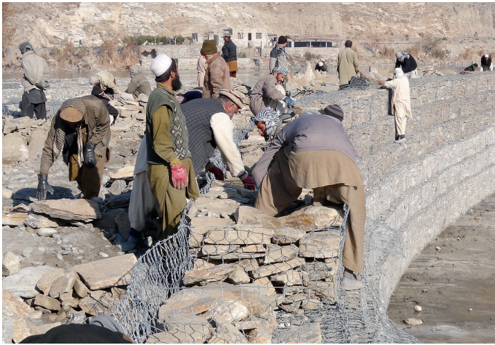
Figure 1.7 Gabion Works at Irrigation Canal 1)
