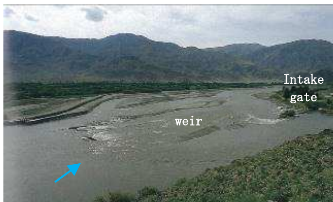
Oblique weir with boulders in the PMS irrigation project (Modeled after Yamada Weir made with traditional Japanese techniques)
