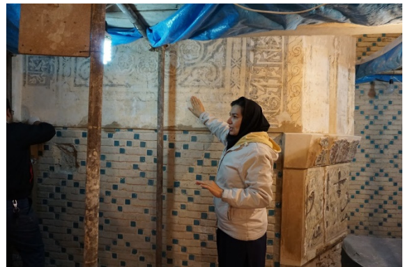
Restoration works undertaken by ICHHTO staff and workers (23/05/19)
