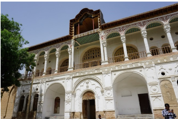
Moshir Diwan Mansion under restoration by ICHHTO (25/05/19)
