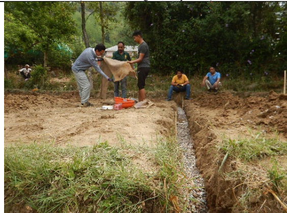
Setting underground drainage (Ragloo, Kangra, April 2022)
