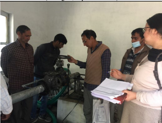
Explanation of operation and function of sluice valve by extension officers using checklist in Motor Pump Training (February 2021)
