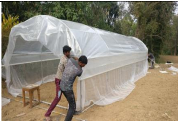
S. No. 3: Walk-in tunnel installation, Chelleli, 15/11/2017
