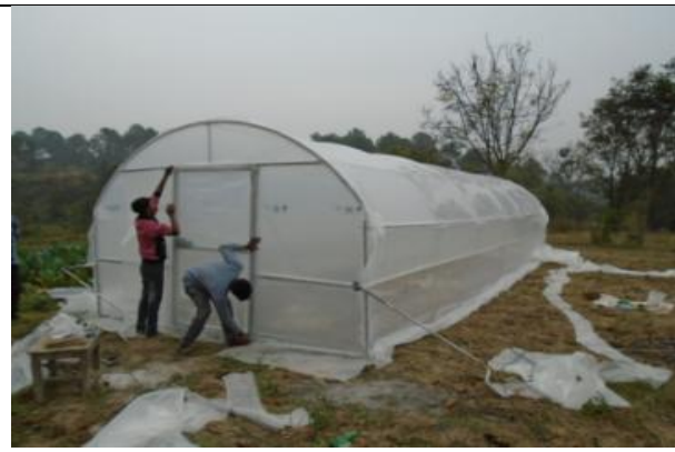
S. No. 4: Walk-in tunnel installation, Balhseena, 16/11/2017
