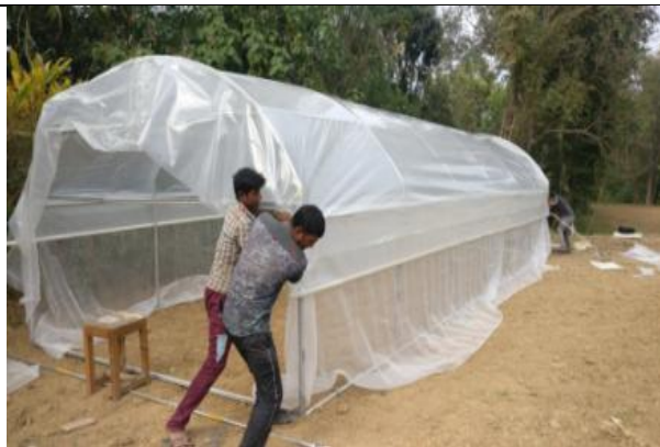
S. No. 3: Walk-in tunnel installation, Chelleli, 15/11/2017
