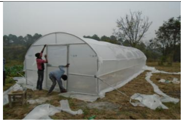
S. No. 4: Walk-in tunnel installation, Balhseena, 16/11/2017
