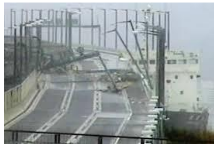
Collision airport access bridge, Osaka, Japan 2018
