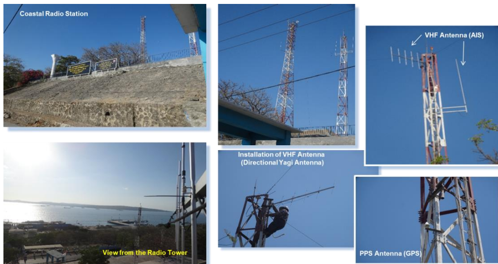
Gambar 5.7 -1 : Installation of AIS Antenna
