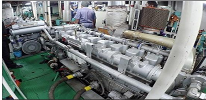
Replaced engine(KN Mina)
