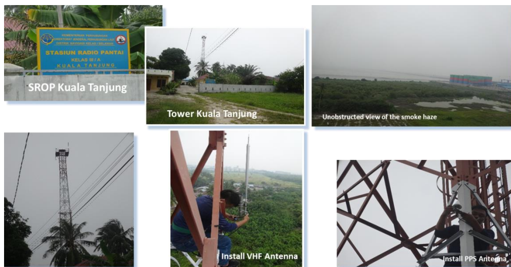
Gambar 5.3 -1 : Installation of AIS Antenna
