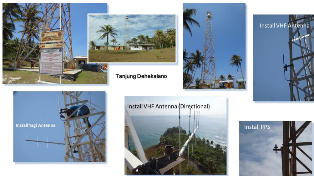
Gambar 5.8 -1 : Installation of AIS Antenna
