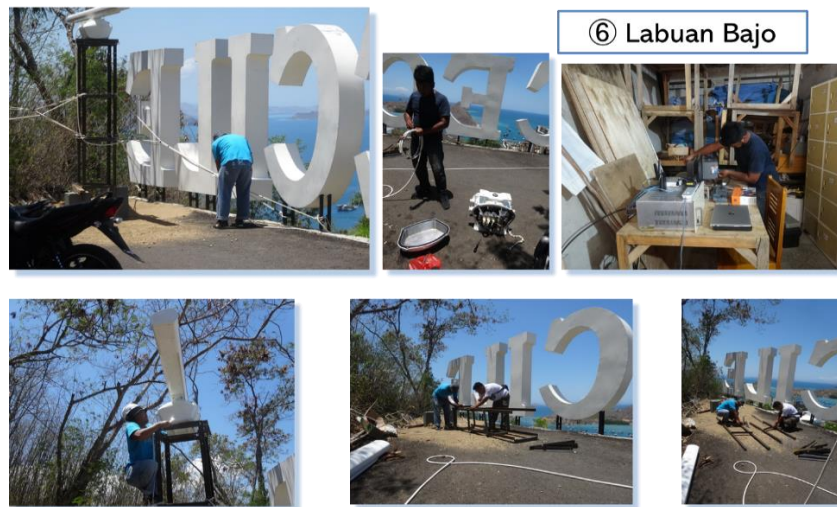
Gambar 5.6 -1 : Installation of Radar
