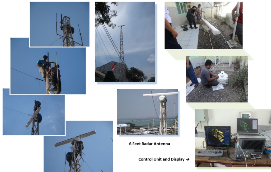
Gambar 5 -3 : Installation of Radar
