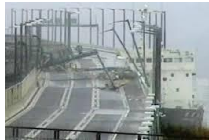
Collision airport access bridge, Osaka, Japan 2018
