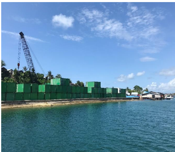
Photo 31 Tual Visit - Container Yard at Tual Port
