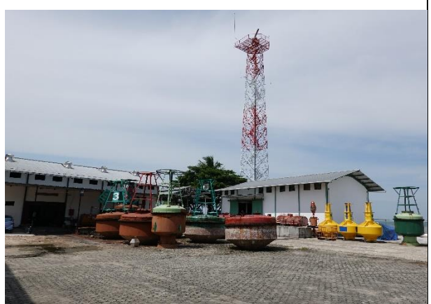
Photo 59 Tarakan Visit - Workshops Facilities
