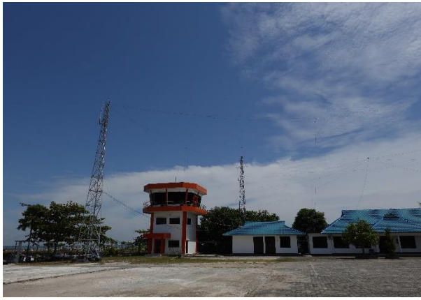
Photo 66 Tarakan Visit - VTS Station
