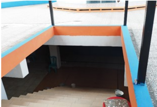
entrance to basement
