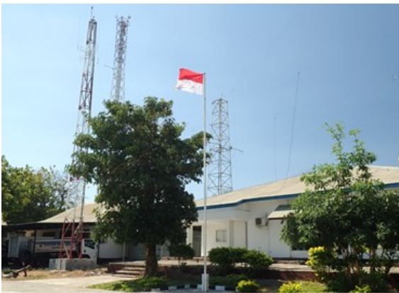
Coastal Radio Station(RX)
