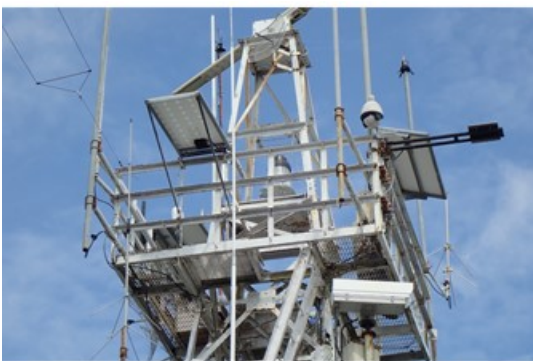
Various kind of Antennas are equipped. Lantern is under the Radar pedestal.
