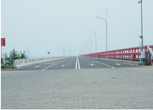
Connecting road to jetty
