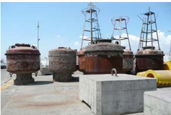
before maintenance body
