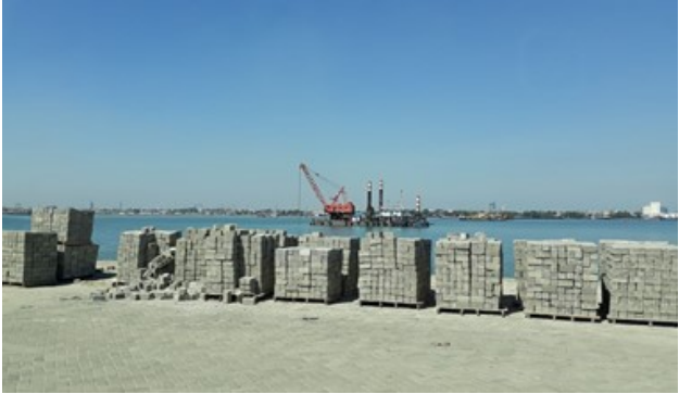
Reventment work and Dredging work
