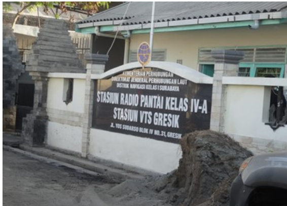
VTS and Coastal Radio Station
