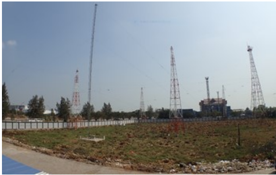
TX antenna group
