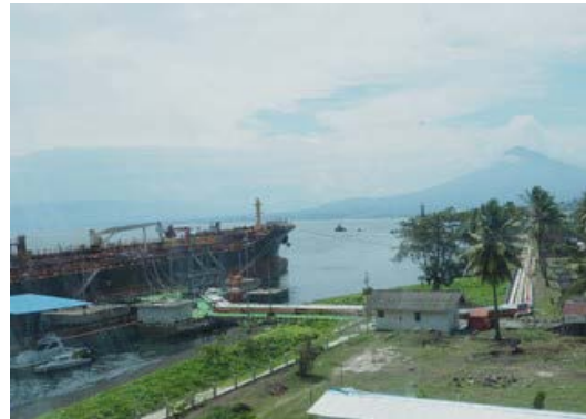
Palm oil loading berth and pipe line
