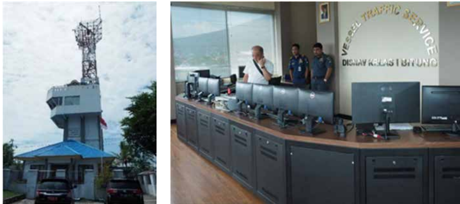
Picture 4.1.11 -3 : Bitung VTS tower, Bitung VTS operation room
