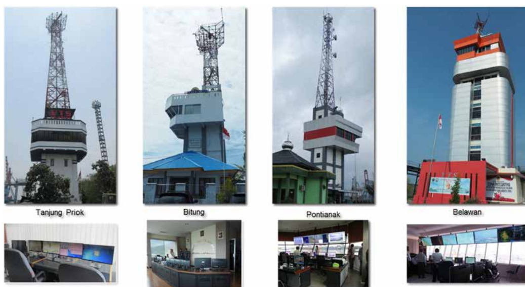
Picture 3.1.4 -1 : VTS Building and Operation Room
