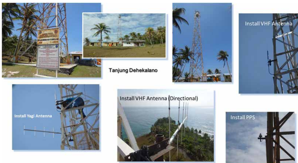
Picture 5.8 -1 : Installation of AIS Antenna
