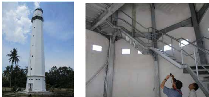
Picture 4.1.10 -5 : Tg. Intan Lighthouse
