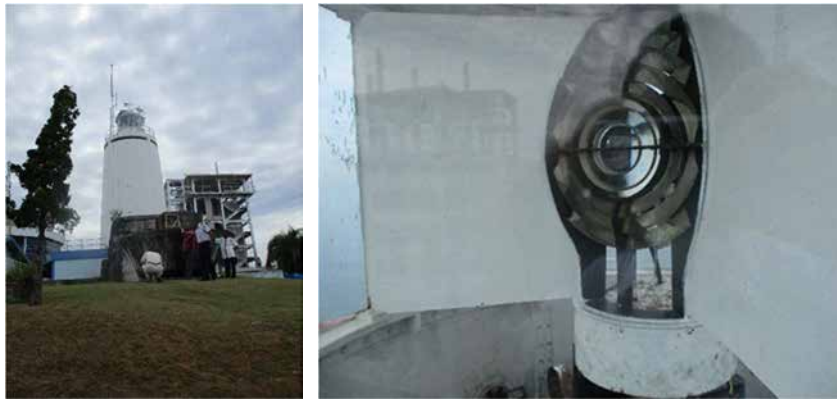
Picture 4.1.13 -6 : Lighthouse structure, Lens part
