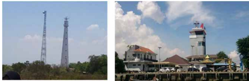
Picture 4.1.12 -1 : Surabaya VTS sensor tower and office
