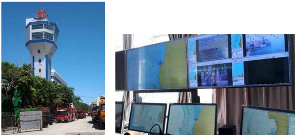
Picture 4.1.7 -1 : Makassar VTS Tower, Displays in Operation Room
