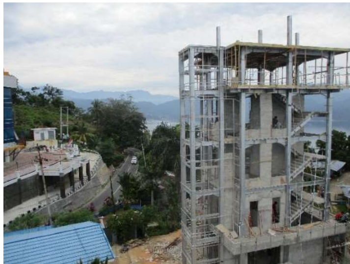
Picture 4.1.13 -7 : New building under construction
