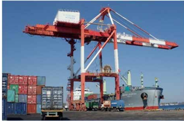
Picture 4.1.1 -1 : Container Yard and Gantry Crane
