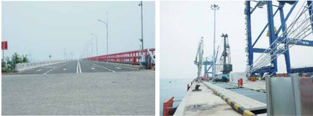
Picture 4.1.8 -5 : 2.8 km Length Jetty, 500 m Length Berth
