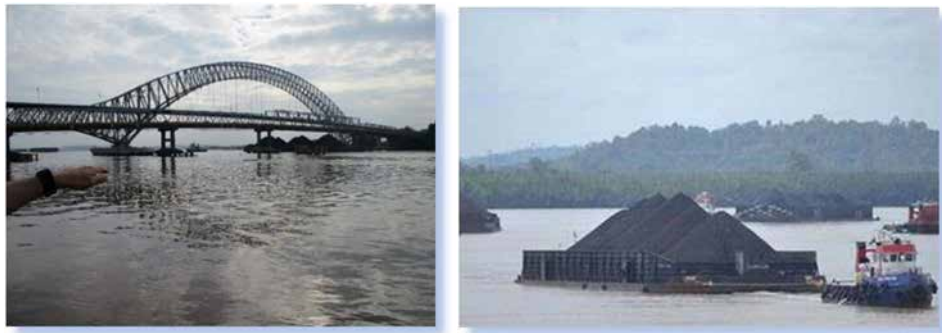
Picture 4.1.5 -1 : Mahakam Bridge, Barge towed by Tug boat
