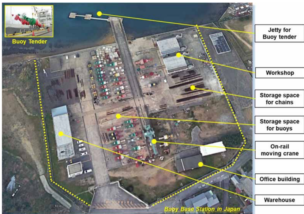
Picture 6.7.1 -1 : Buoy Base Station in Japan
