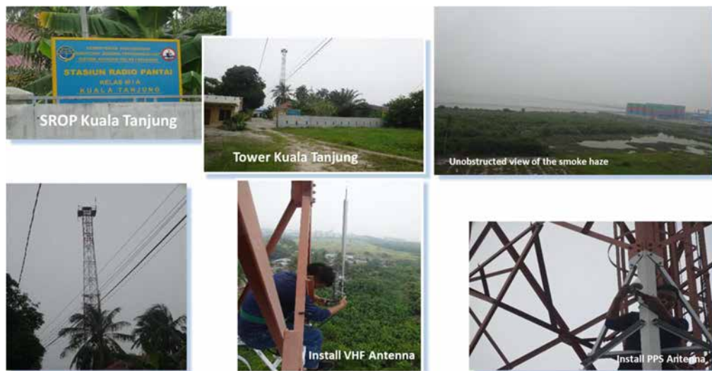
Picture 5.3.-1 : Installation of AIS Antenna
