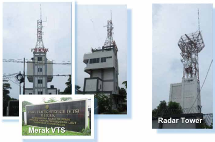
Picture 5.9 -1 : Merak VTS and Radar Tower
