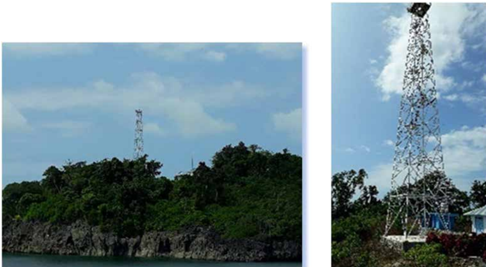
Picture 4.1.3 -6 : Tg. Burang Lighthouse
