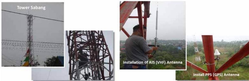
Picture 5 -2 : Installation of AIS and GPS Antenna
