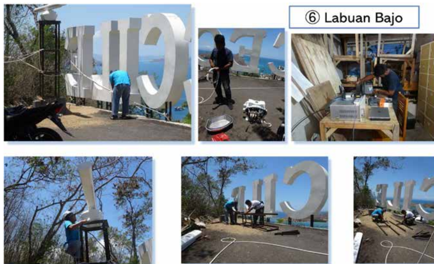
Picture 5.6 -1 : Installation of Radar
