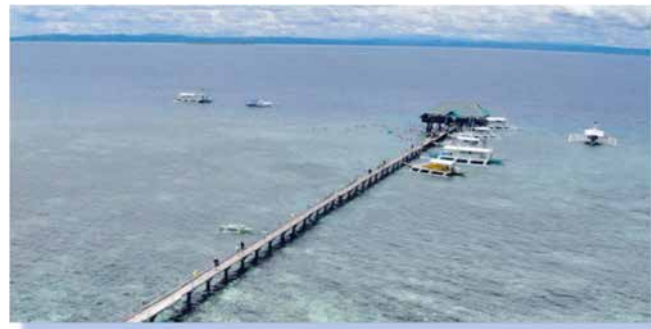
Figure 6.4.2 -7 : Sector Light at Tip Point of Pier
