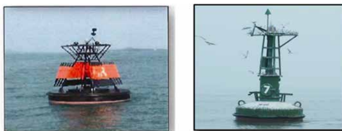
Picture 3.1.1 -3 : Floating Lighted Buoy
