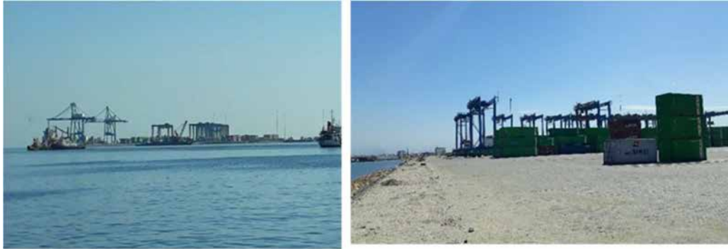
Picture 4.1.7 -4 : Gantry Crane, Container Storage Yard
