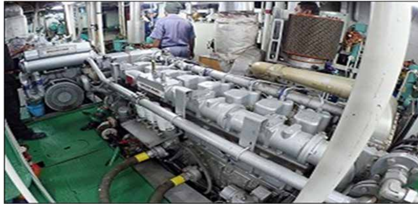
Replaced engine(KN Mina)
