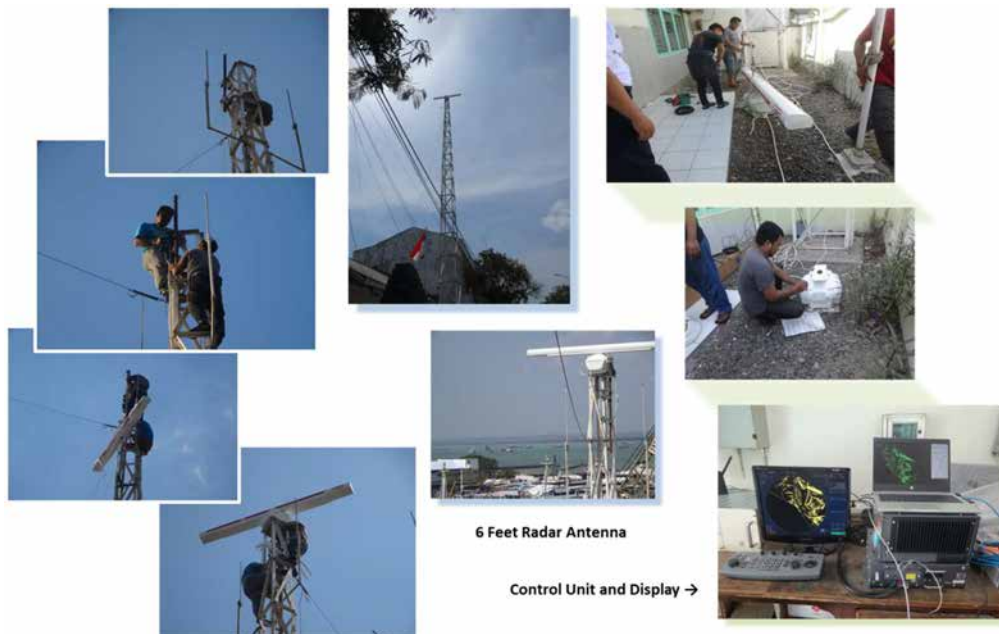
Picture 5 -3 : Installation of Radar
