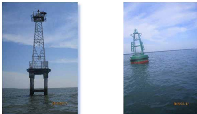
Picture 4.1.6 -4 : Lighted Beacon, Floating Buoy
