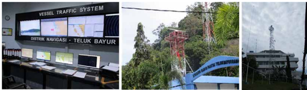
Picture 4.1.13 -4 : Facilities of VTS
