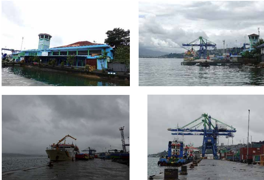
Picture 4.1.2 -5 : Port of Ambon
