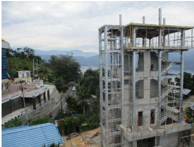
第 4. 1. 13 -7 写真 New building under construction
