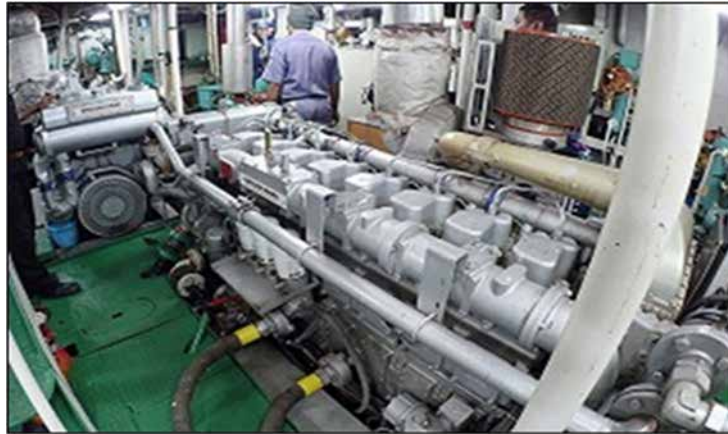
Replaced engine(KN Mina)
