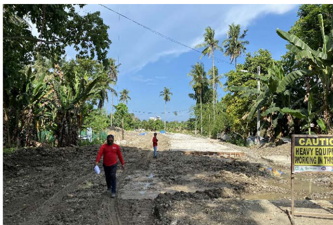
Widening construction section
