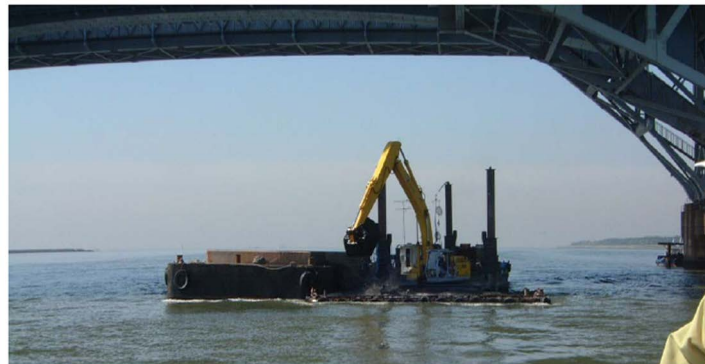
Figure 4.4.14 Image of Backhoe Dredging
