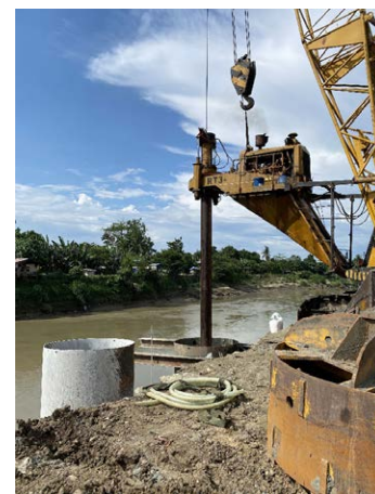
New construction section
