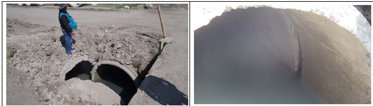
Figure 2.9.9 Example of Inadequate Connection of Pipes
