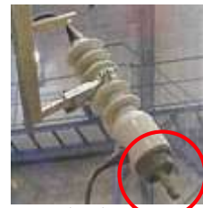
Source: NGK Insulators, Ltd.
