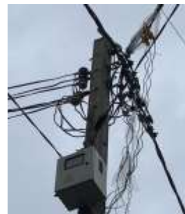
VI measurement instruments in a box on pole in a rainy day
