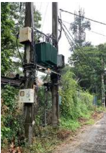
VI measurement instruments in a box on pole in a rainy day
