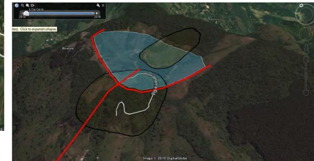
Upper reservoir and Possible landslide (black line)
