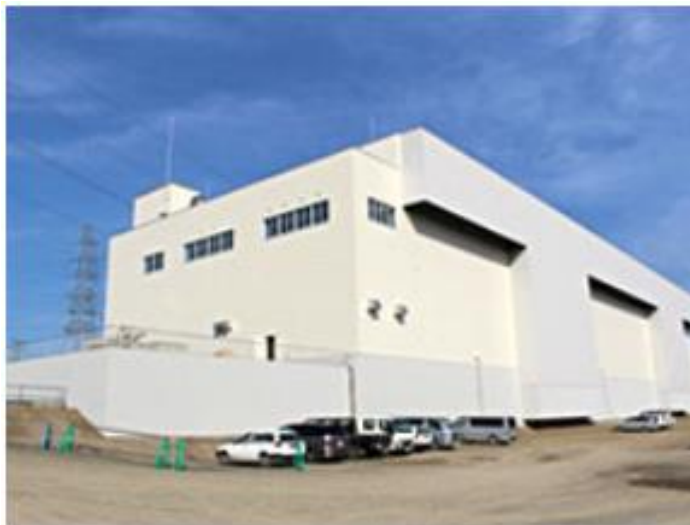
Exterior view of storage battery building
