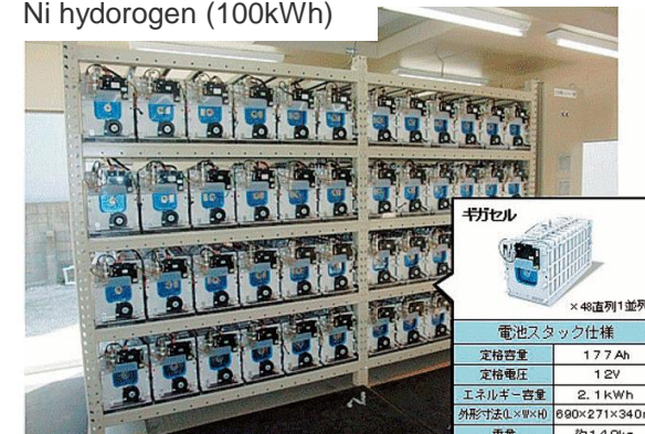
Ni hydrogen (100kWh)
