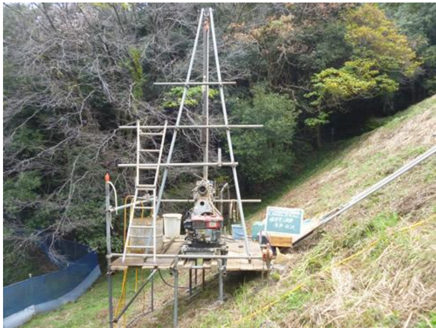
Core Drilling at site
