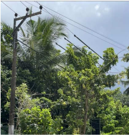
Installation of ARC
