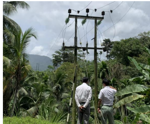
Confirmation and OJT of OCI installation
