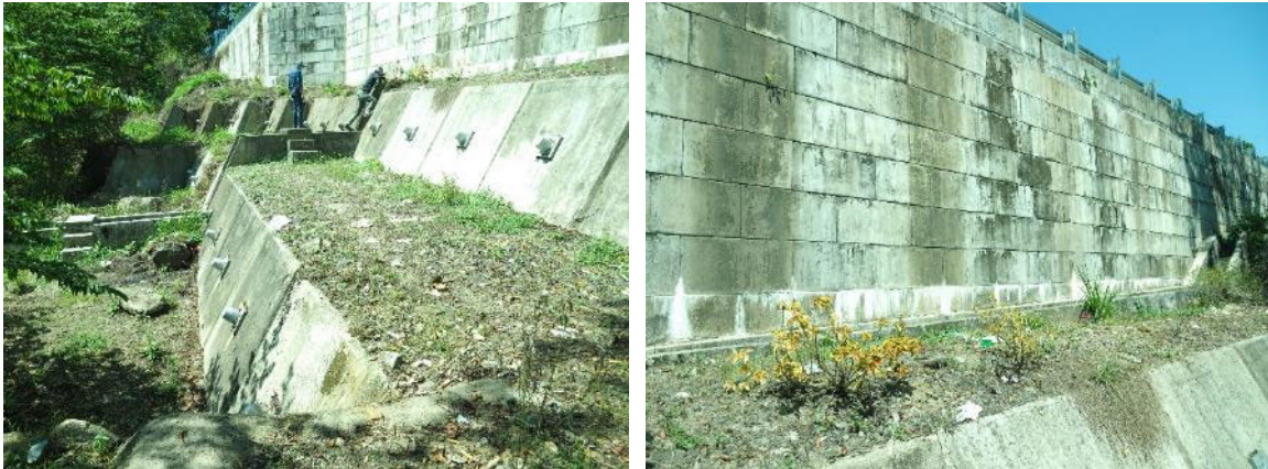
Figure 5-3 Anchor Works and Light Embankment Works by LDPP
