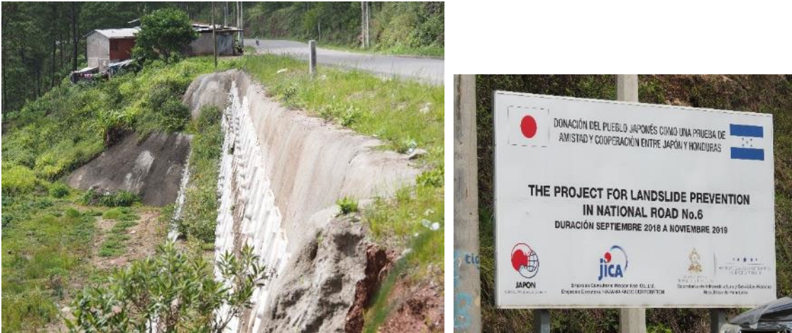
Figure 5-7 Landslide Countermeasure along National Highway No. 6 (Sta.14.7km)
