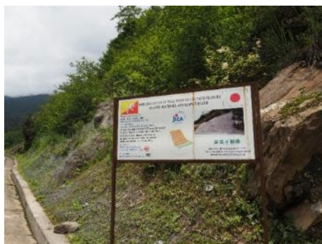
Macro net construction method signboard
