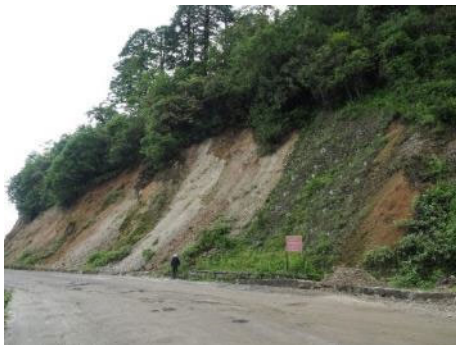
The test construction site of non-frame
