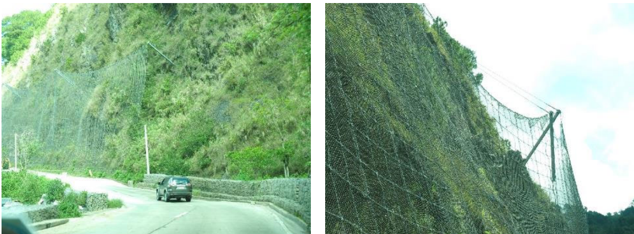
Figure 5-4 Pocket-Type Rock Fall Protection Net Constructed under a JICA Project
