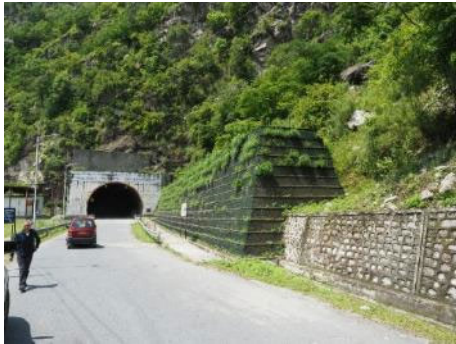
Rock fall protection embankment in front of the tunnel entrance
