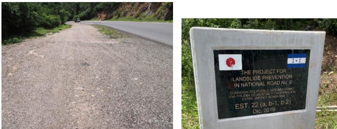
Figure 5-8 Landslide Countermeasure along National Highway No. 6 (Sta.22km)
