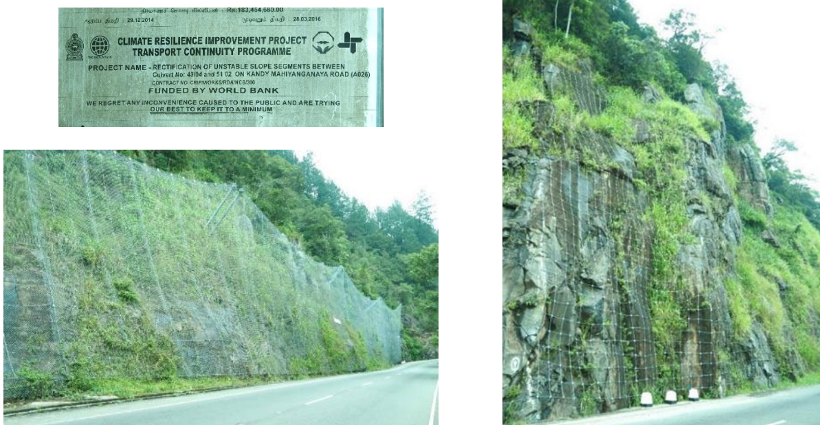
Figure 5-1 Japan's Rock Fall Countermeasures Constructed by the World Bank's Project
