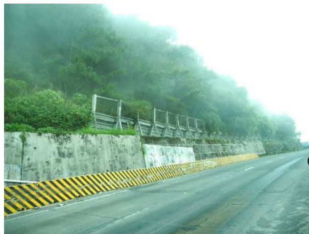
Figure 5-6 Rock Fall Protection Fence on Rosario-Pugo-Baguio Road
