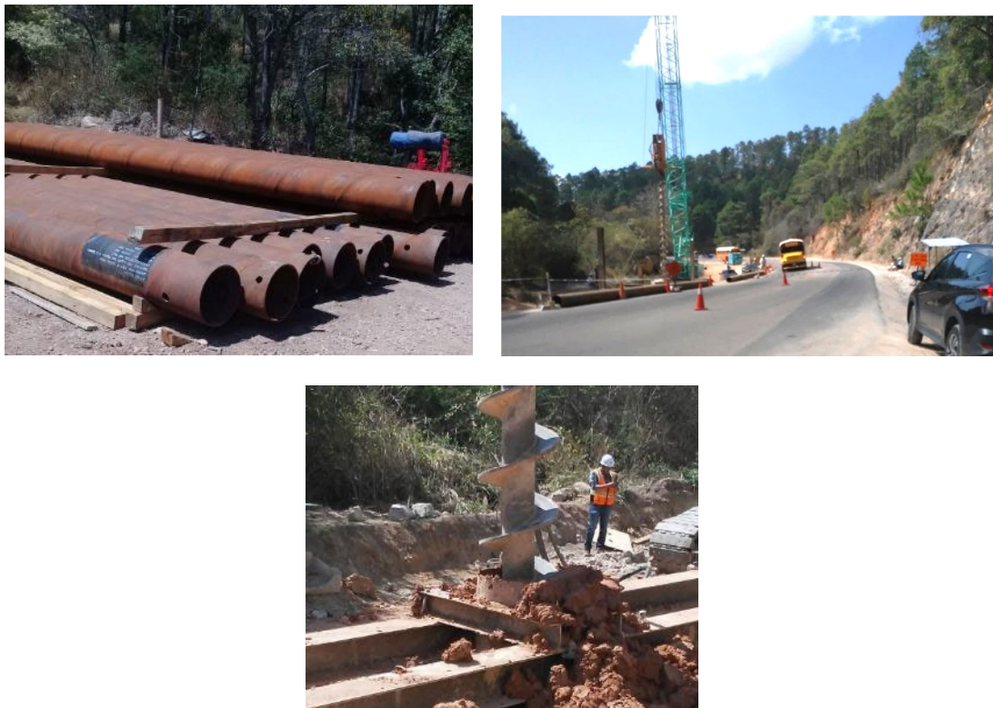
Figure 5-9 Construction of Steel Pipe Piling in 2019
