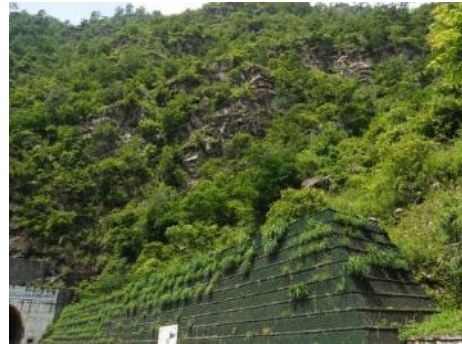
Rock slope behind rock fall protection embankment
