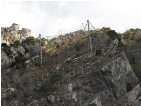
Rock fall fence (France)
