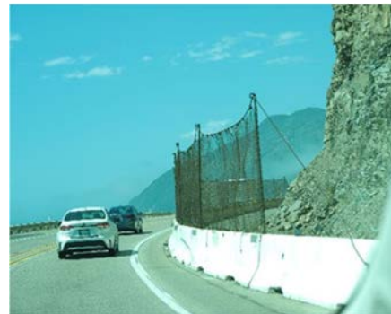
Pockets secured by concrete blocks with simple fence.
