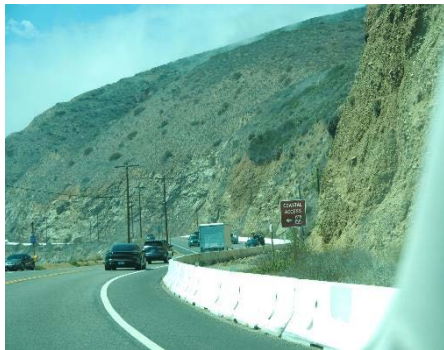
Pockets secured by concrete blocks.
