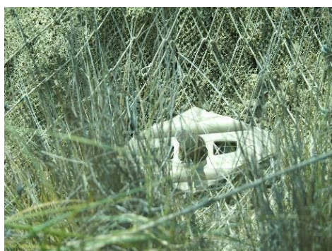
Cable net with rock bolts/nailing
