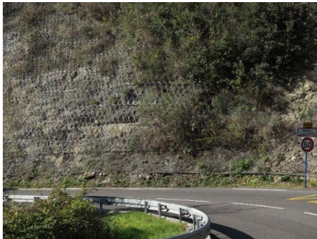
Cable net with rock bolts/nailing (France)
