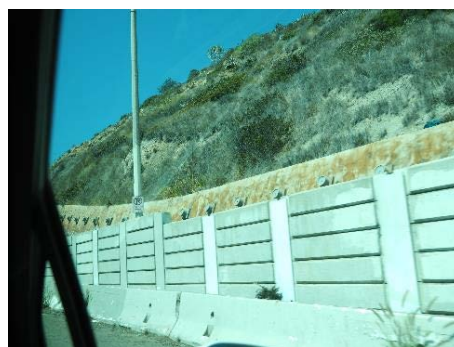
Retaining wall with ground anchors
