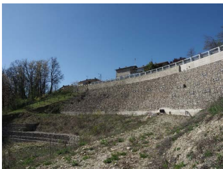
Gabion with nailing (Italy)
