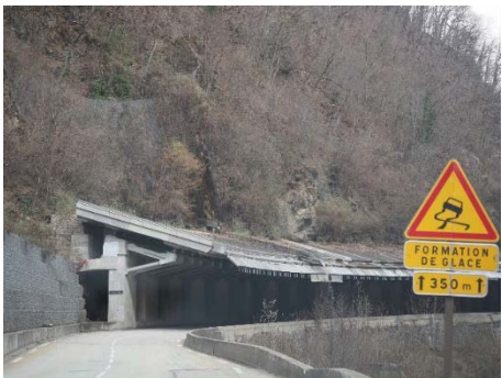
Rock shed (France)
