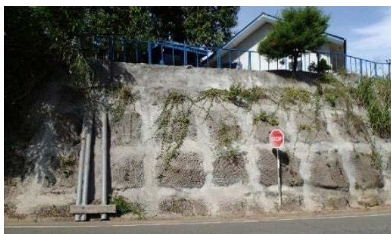
Example of embedded crib works that has been implemented since 2000s
