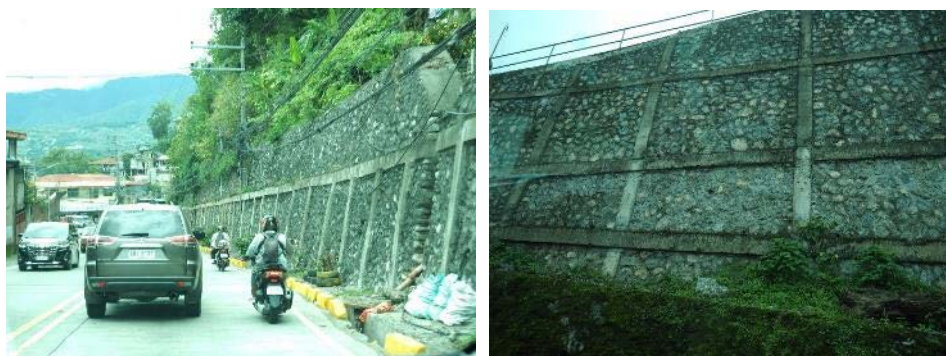
Figure 5-2 Example of Masonry Retaining wall with Cast-in-situ Concrete Crib Works
