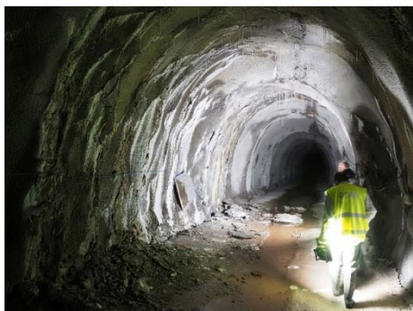
Drainage tunnel at San Lorenzo Tunnel
