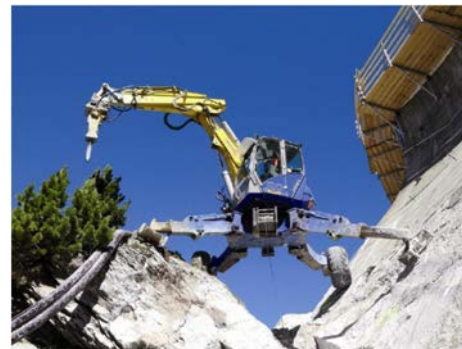
Work on rock slope.
