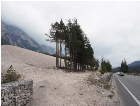
Debris flow merlon along the highway
