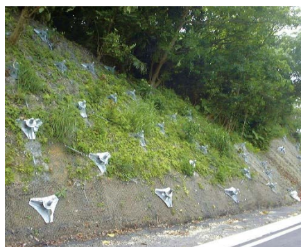
(a) Non-frame construction method
