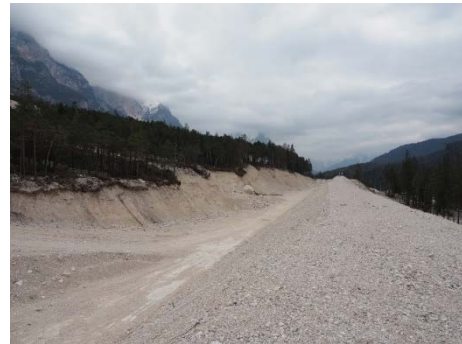
Pockets to trap debris flow behind merlon
