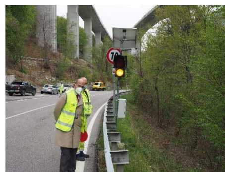
Signal connected with EWS (Italy)
