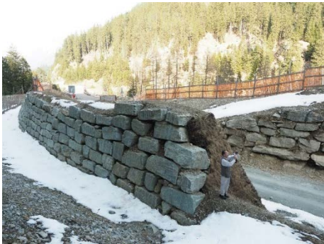
Rock fall merlon which can endure fallen rocks of a weight of 1t hitting at 200km/h. (Switzerland)
