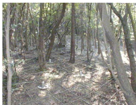
(b) Rope net and rock bolt combination method
