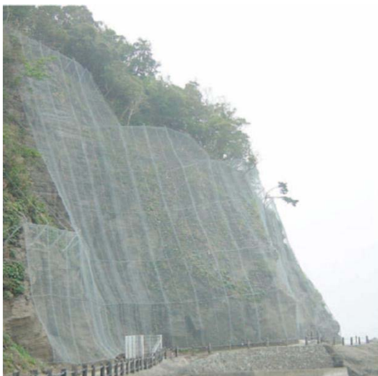
(a) Conventional Pocket-type Rock Fall Net
