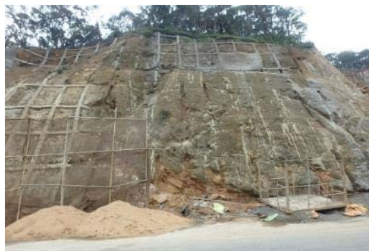
Figure 5-9 Cast-in-situ Concrete Crib Works (Excavated Type) in Sri Lanka
