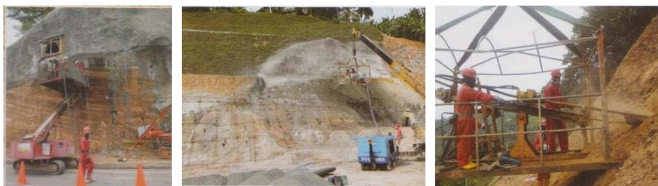
Figure 5-14 Two Types of Platform with Heavy Machinery in Sri Lanka
