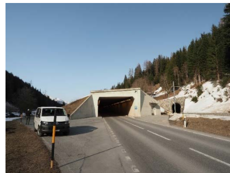
Debris flow cum snow avalanche shed
