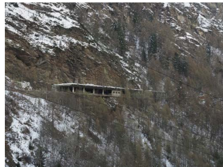
Rock shed (Switzerland)
