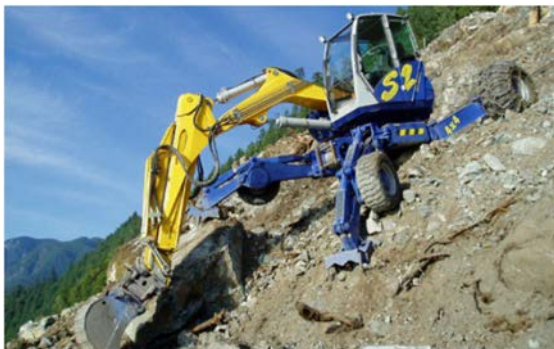
Work on steep slope.
