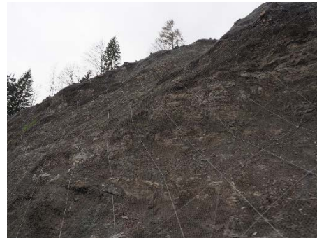
Net and cables with rock bolts/ nailing (Italy)
