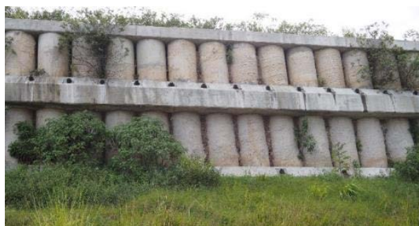
Figure 5-10 Continuous Pile Retaining Wall Combined with Anchor in Honduras
