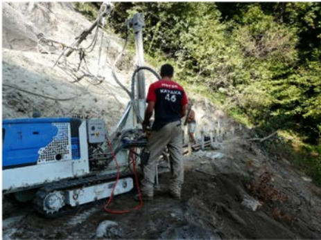
Machinery for micropile installation.
