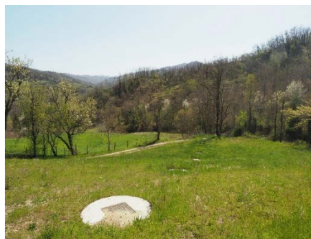
Top concrete ceiling of small diameter drainage wells
