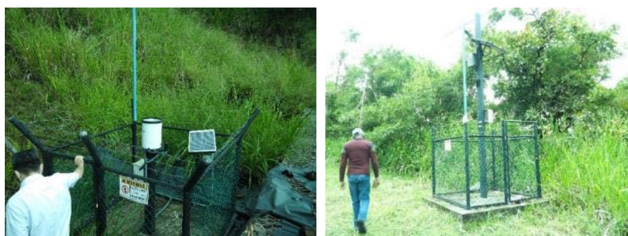
Figure 5-15 Rainfall Observation Instruments at Landslide Site in Sri Lanka
