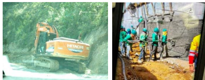
Figure 5-12 Road Widening in Philippines (left) and Spraying Work in Honduras (right)
