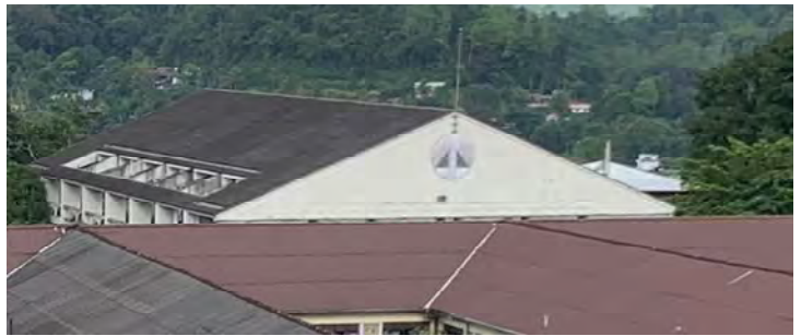
JICA Building (パネル設置)
