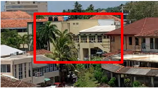
Accident & emergency (パネル設置)
