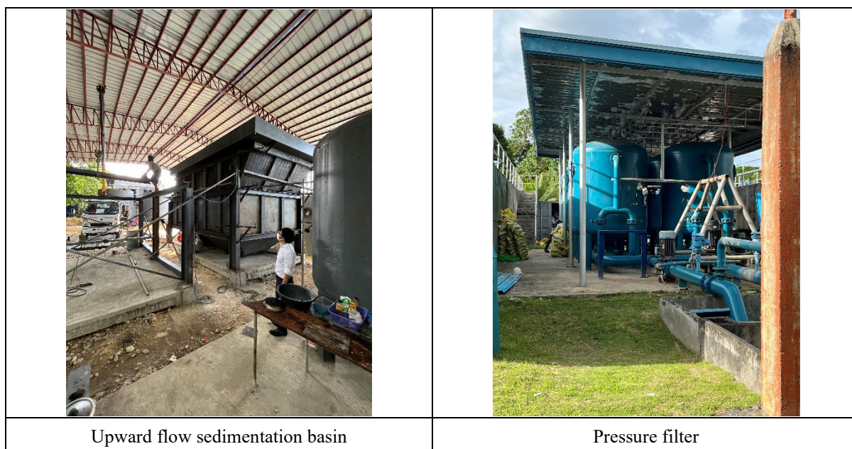
Photo 7-2-1 Expansion WTP Under Construction
