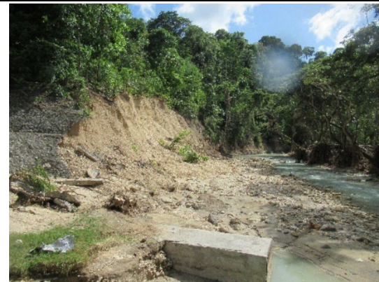
(Photo-4) Partial Collapse of Dimapatoy River Bank after passing Typhoon Paeng
