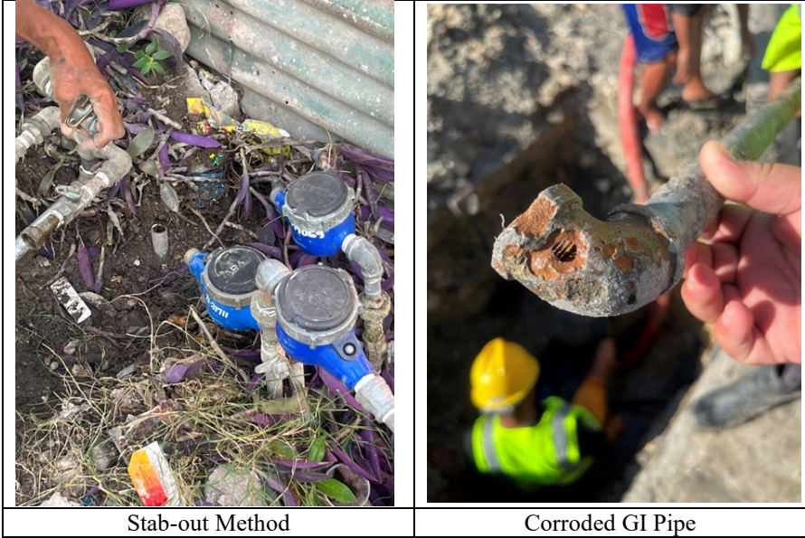
Photo 2-4-1 Leakage Repair
