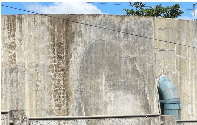
Photo 2-4-2 Degraded Condition of Concrete Structure
