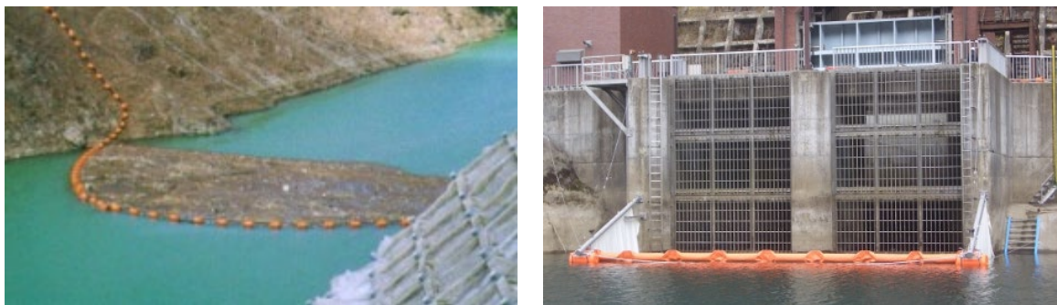
Photo 6-3-3 Installation of Floating Nets at Gate Facilities
