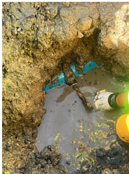
Photo 2-5-1 Horizontally Drilled Saddle
