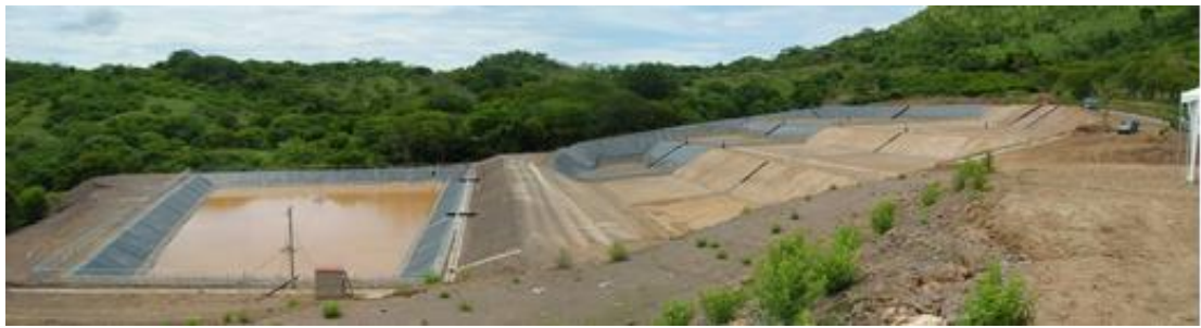
Photo 7-26 Newly Constructed Sanitary Landfill (Phase 2)
