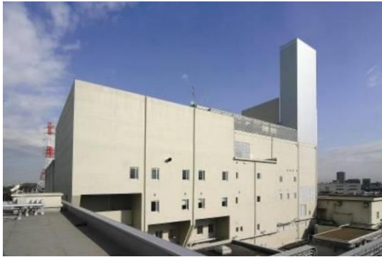
Photo 6-17 North Incineration Plant (150t/24h×1 unit)
