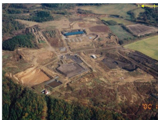
Photo 5-7 Overview of Illegal Dumping (2000)
