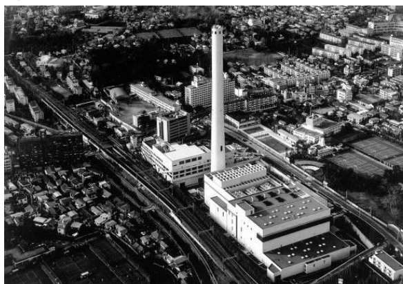
Photo 6-8 Sugunami Incineration Plant
