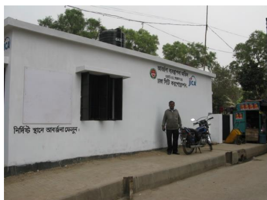
Photo 7-41 Ward Cleaning Office
