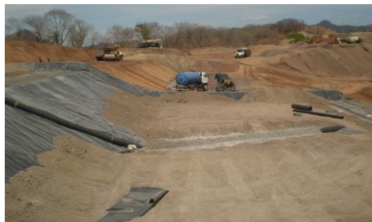
Photo 7-17 Sanitary Landfill under Construction (Phase 2)
