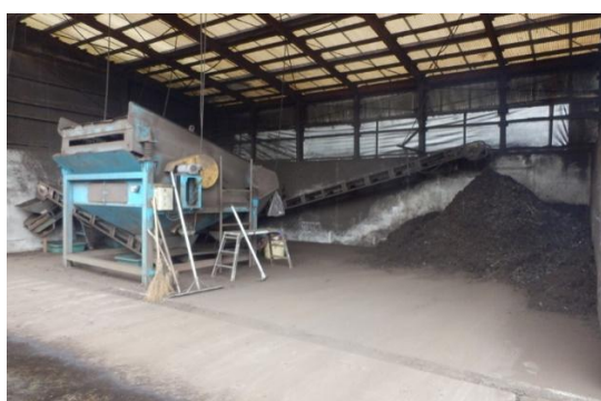
Photo 6-34 Final Processing Process after Maturing
