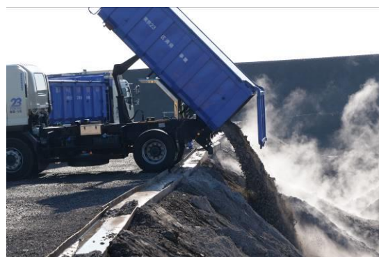
Photo 6-15 Landfill of Incinerated Ash
