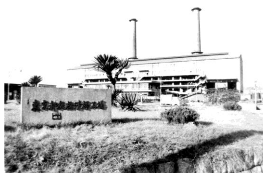
Photo 6-4 Itabashi Incineration Plant (Completed in 1961)
