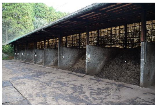
Photo 6-31 Concrete Composting Yard
