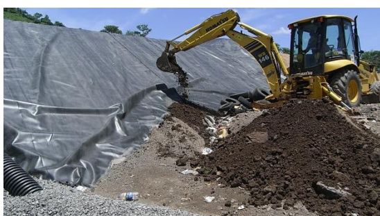
Photo 7-18 Practice of Applying Soil Cover
