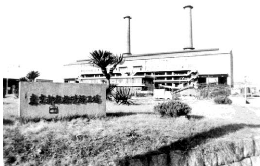
Photo 19 Itabashi Incineration Plant (Completed in 1961)
