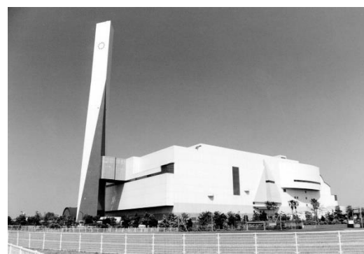
Photo 4-28 Shin-Koto Incineration Plant (Completed in 1998)
