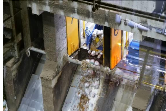
Photo 4-35 (1) Platform (Waste Pit)
