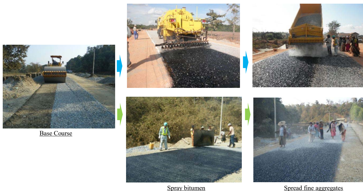
Figure 1-11 Construction Procedure of Bituminous Surface Treatment
