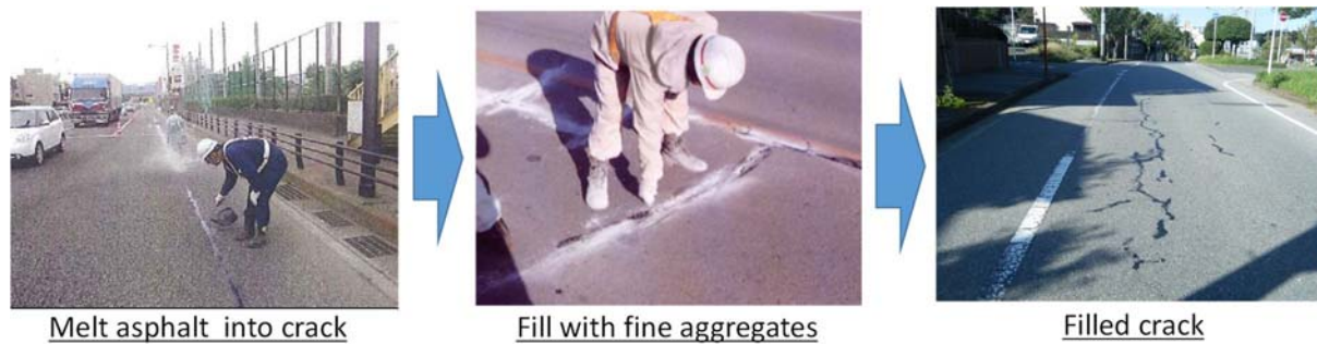
Figure1-4 Road Maintenance with Filling Port Hole
