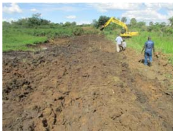
Embankment work around swamp area
