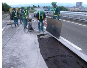
Spray bitumen (e.g. Tack coat)
