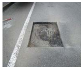
Remove damaged area
