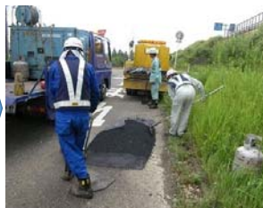
Pave with mixed asphalt material
