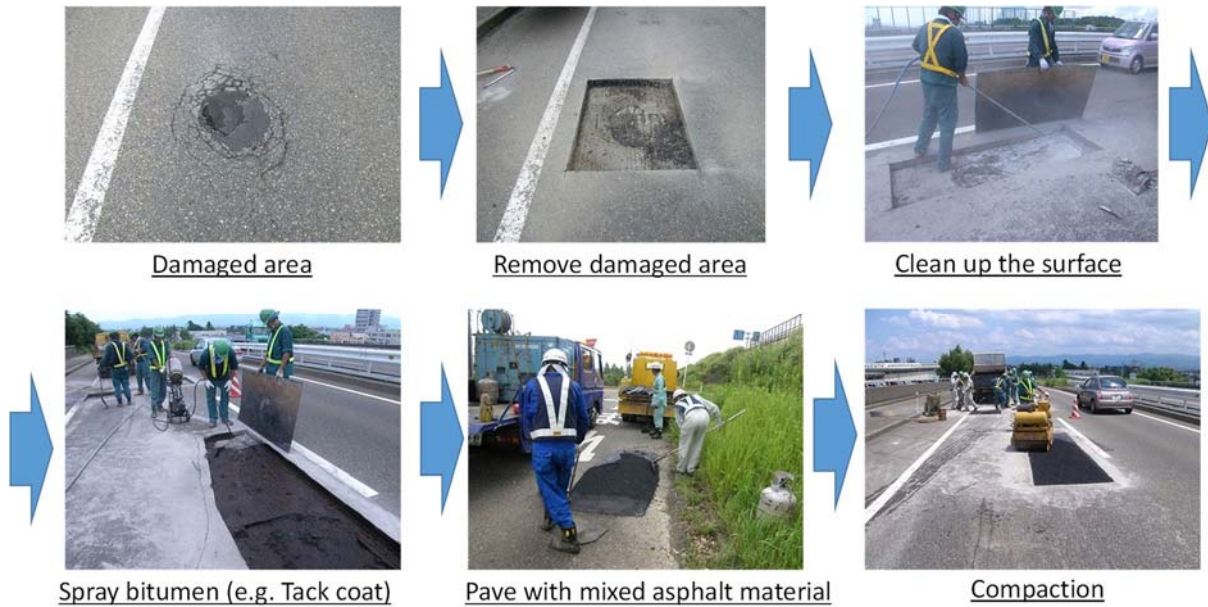
Figure1-4 Road Maintenance with Filling Port Hole
