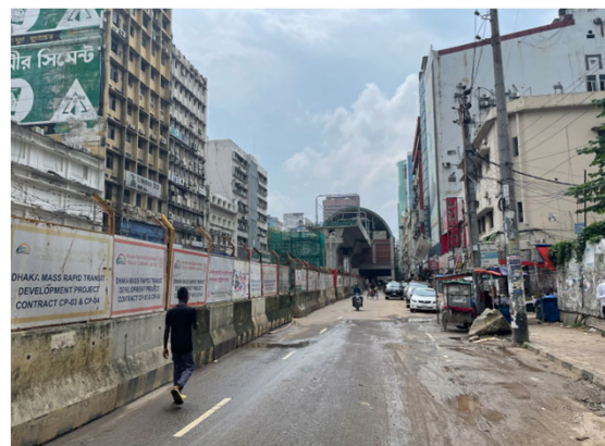
Source: JICA Expert Team Construction site at Motijheel station (Kamalapur side)
