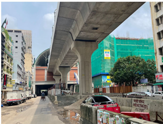
Source: JICA Expert Team Motijheel station (Agargaon side)
