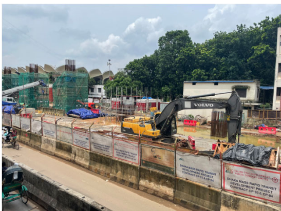
Source: JICA Expert Team Construction site at Kamalapur station
