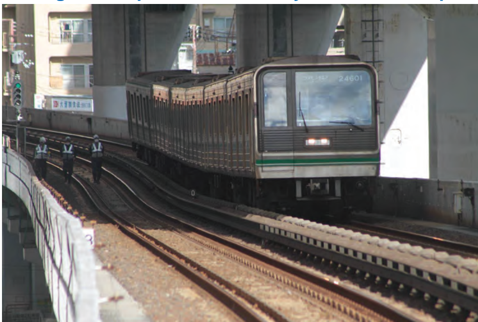
Photo 1: Patrols and Inspections during Operating Hours What dangers and potential risks do you think in this picture?
