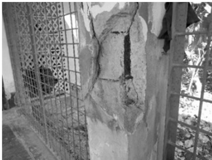
Beams in the Corridor of the Education Building Govt. TTC Rajshahi
