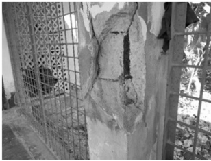
Beams in the Corridor of the Education Building Govt. TTC Rajshahi
