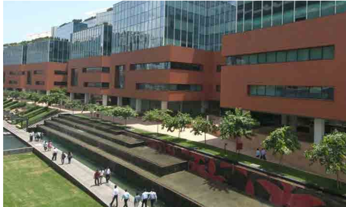
13. Office buildings clustered around landscape public spaces
