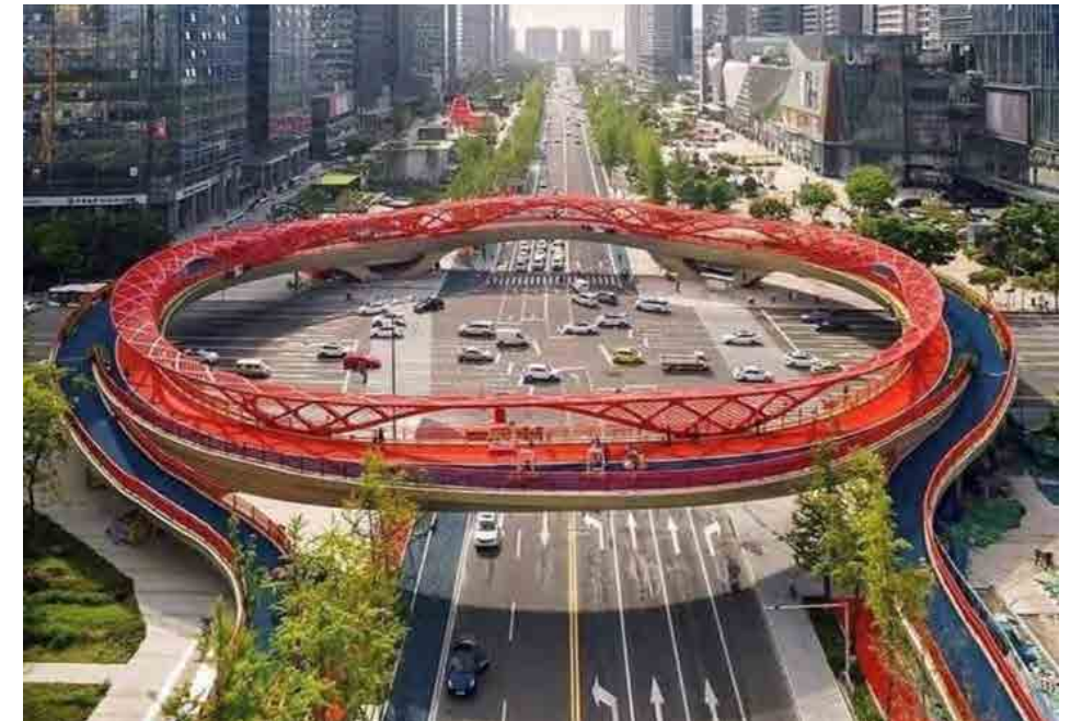
10. Landmark elevated walkway ring ( Ring of Jiaozi, China )
