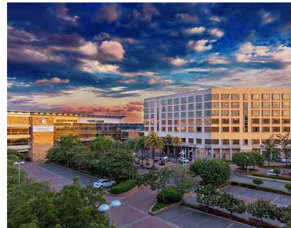
8. Hotel & Convention Center (Source: Paya Lebar Quarter (Station area TOD) Singapore)
