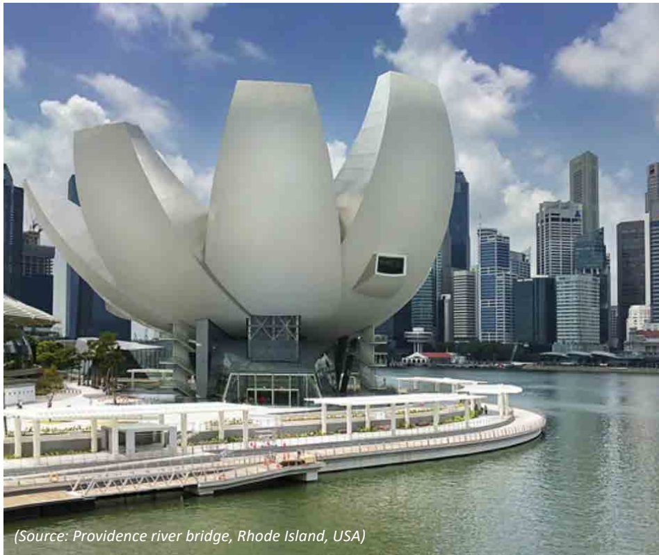
11. Landmark convention building
