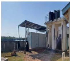
Vanga fish landing site with solar-powered cold store and dice plant
