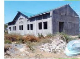
Malindi fish landing site under construction
