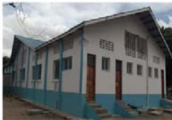
Ngomeni fish landing site, has a fish market, cold store and ice plant
