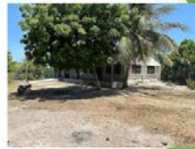
Kipini landing site with ice plant and cold store
