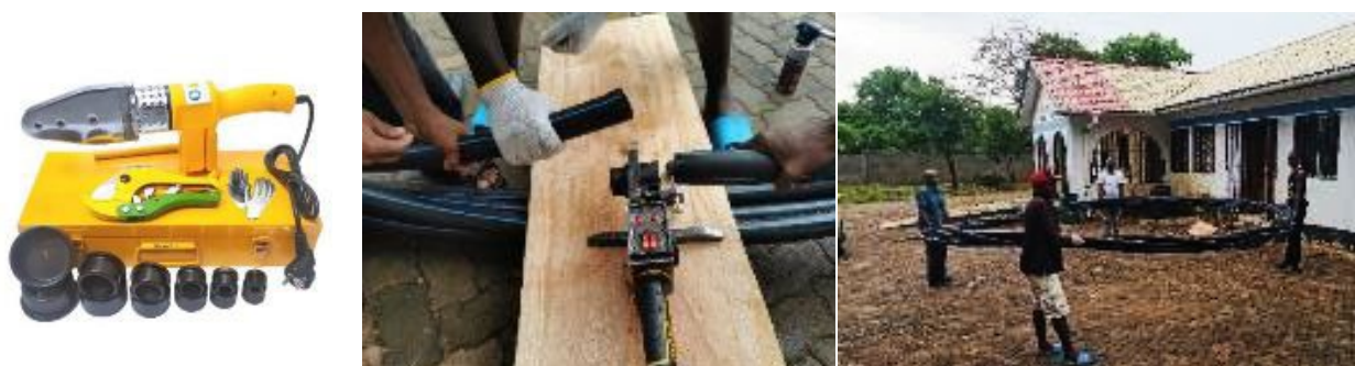
Figure 56. Construction of a small fish cage frame (5m diameter) made with 50mm HDPE pipe using a socket fusion
