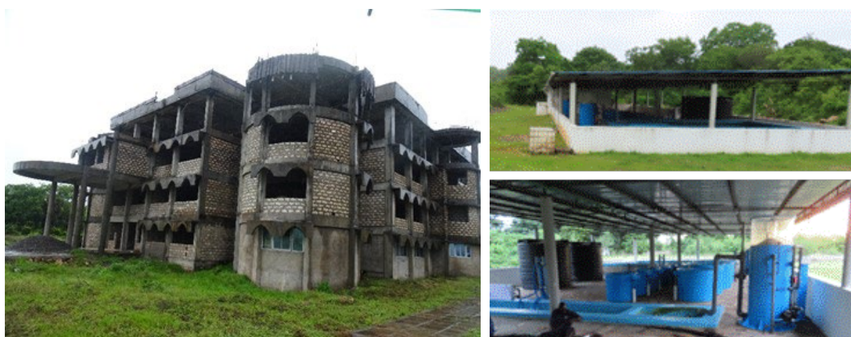
Figure 3. National Mariculture Resources and Training (NAMARET) at Shimoni, Kwale County Main building under construction (left) and Hatchery partially opened (right)
