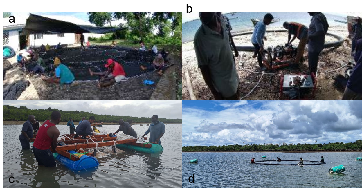
Figure 51. Construction and installation of HDPE fish cage at Shimoni, Kwale County Sewing of fish cage net (a), Butt-fusion welding of HDPE pipes (b), Dropping of concrete anchor blocks (c), and Installation of fish cage in the grid mooring system (d)
