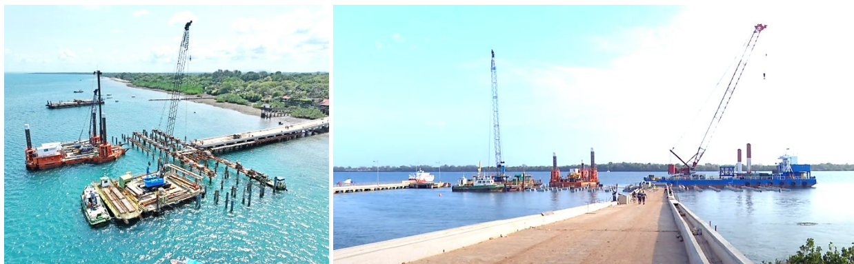
Figure 6. Shimoni Port Jetty Under Construction
