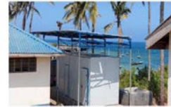
Mayungu fish landing site, cold store and ice plant
