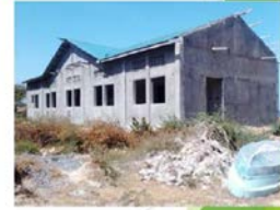
Malindi fish landing site under construction
