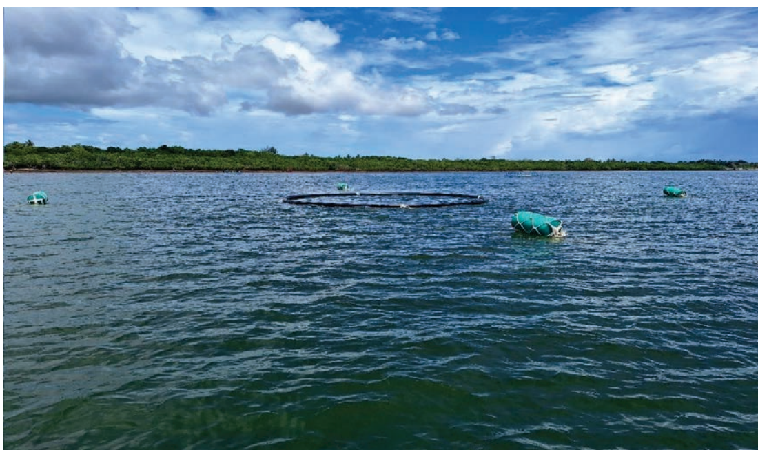
Actual photo of installed HDPE cage with grid mooring system in Kijiweni
