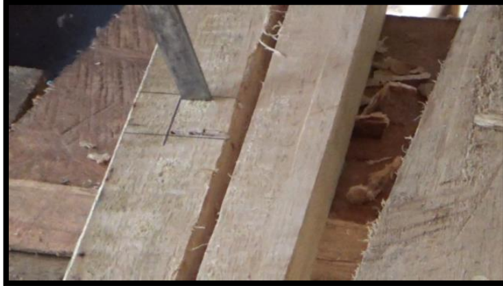
Figure 16. Using a pencil mark the lumber and carve it at which it intersects with each rib.
