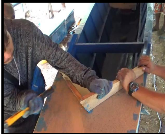
Figure 21. Constructing of barko-barko in Bow area.
