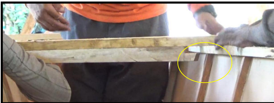
Figure 19. The ends of the braces were trimmed to fit for attaching to the gunwale.
