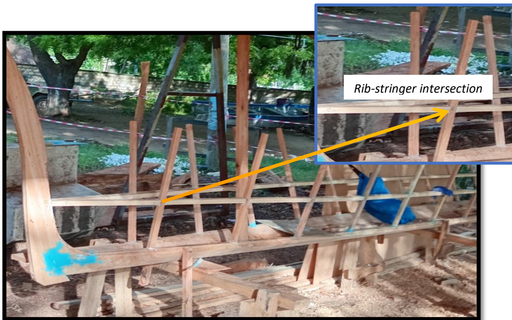
Figure 11. Fastening half lap of stringer at every intersection of the frame with epoxy.
