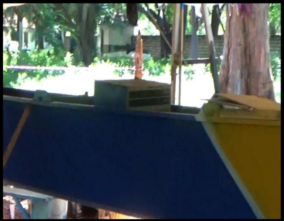
Figure 22. Constructing cover engine.
