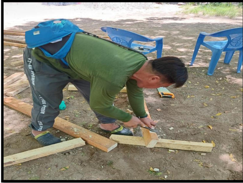
Figure 7. Preparing the 30-pieces ribs.
