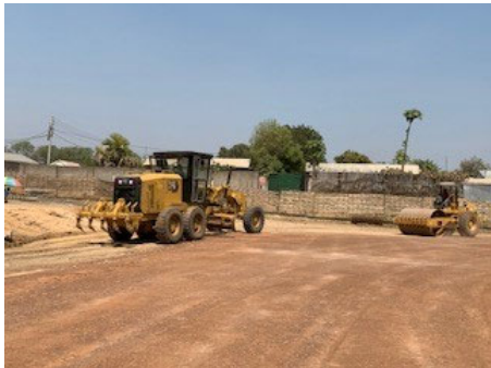
Bulk Ground grading (8th NUD)
