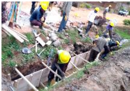
Figure 9.6: Examples of formwork
