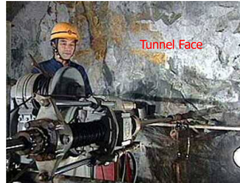
a) Drilling Survey (Horizontal)
