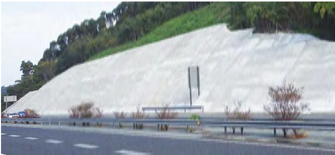
Photo-3 Shotcrete http://green-eng.com/projects/hukitsuke.php
