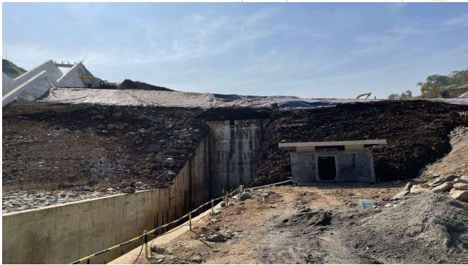
Embankment during wet season
