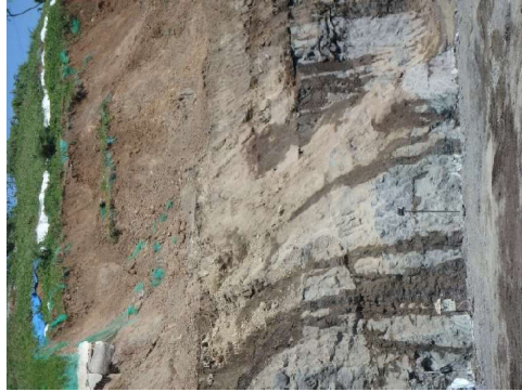
Weathered Basalt on Cut Slope and Collapse in the Soil Layer
