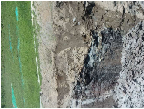
Weathered Basalt on Cut Slope and Collapse in the Soil Layer
