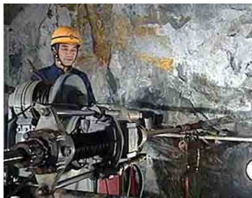
Figure 2.34 Drilling Survey (Horizontal)
