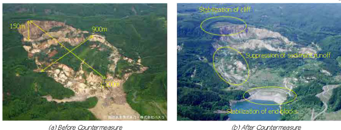
Figure 2.8 Large-scale Landslide in the Dam Reservoir in Japan
