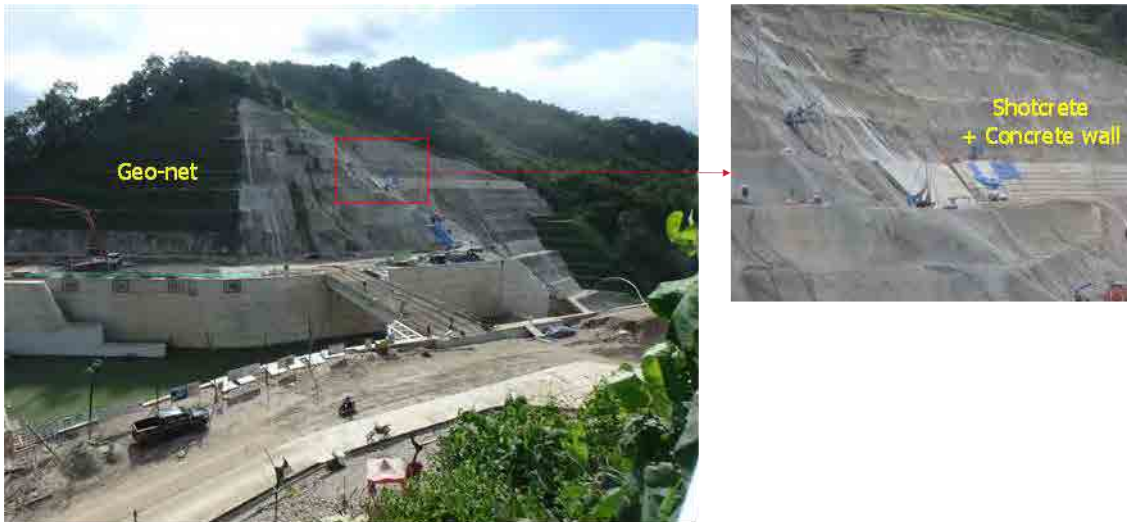
Figure 2.33 Construction of Countermeasures based on Geotechnical Observations (Ameroro Dam)
