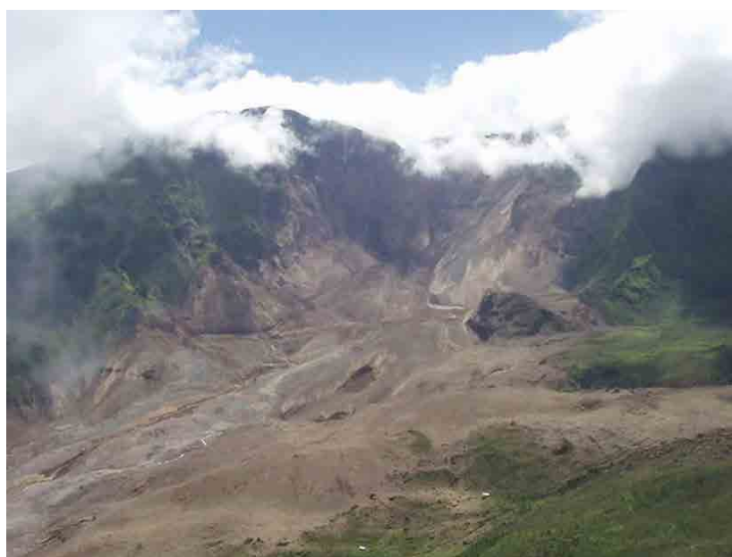
Figure 2.9 Large-scale Landslide in the Upstream of Bili-Bili Dam (2004)
