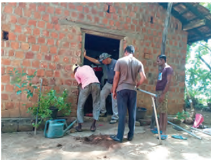
Installation work for handrail at the entrance of residence
